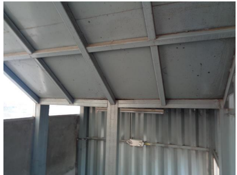
Onsite condition (Middle beams are LB3)
