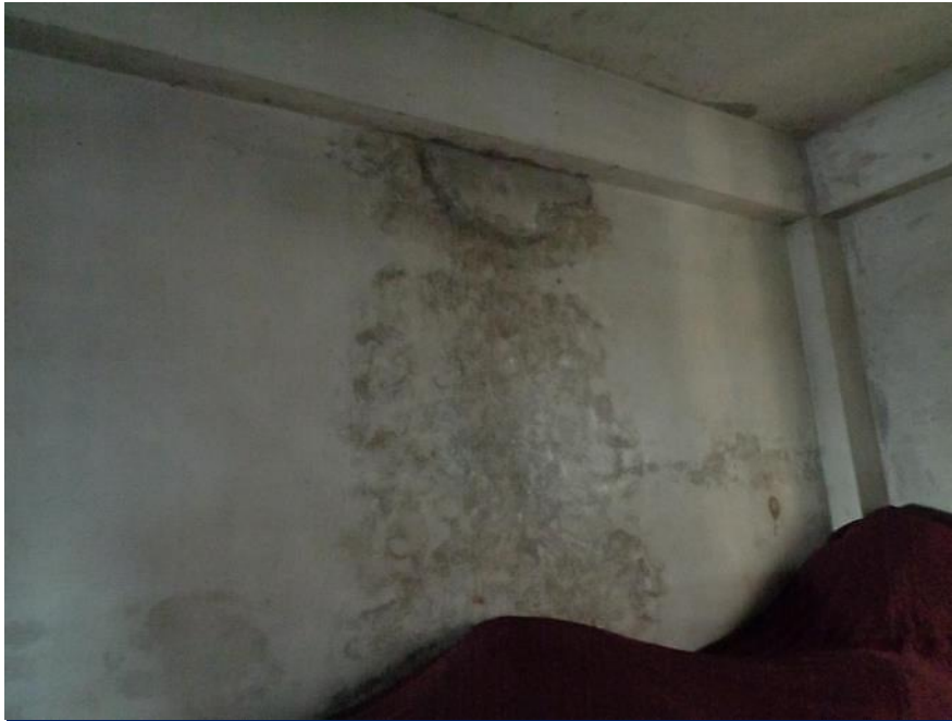
Dampness on wall of RC stair zone
