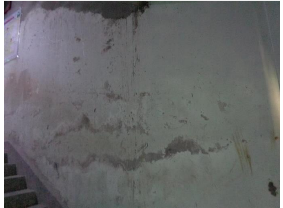
Dampness on wall of RC stair zone
