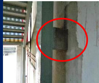
Support to stair
