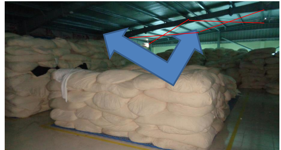
Bracing location shifted
