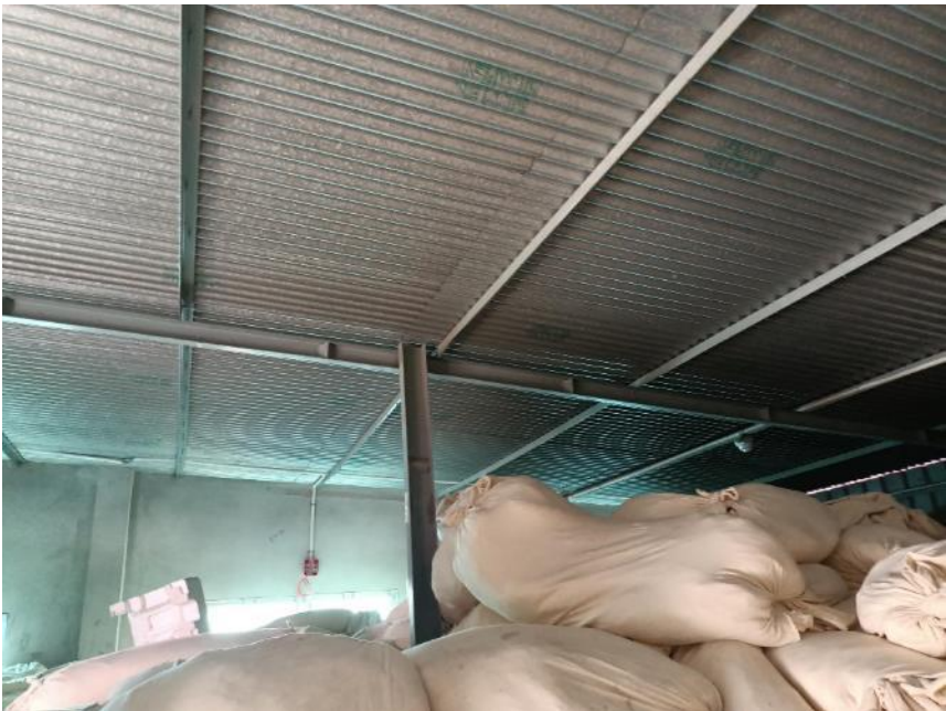
Apparently inadequate connection
