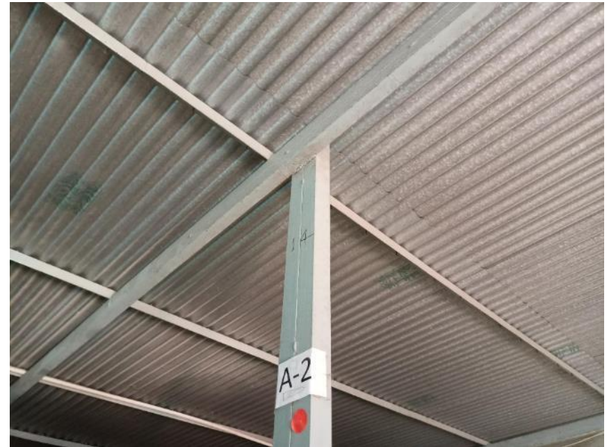
Apparently inadequate connection
