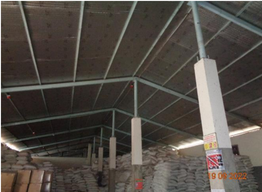
Load transfer media is missing at along long direction
