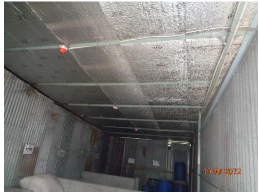
Apparently inadequate connection
