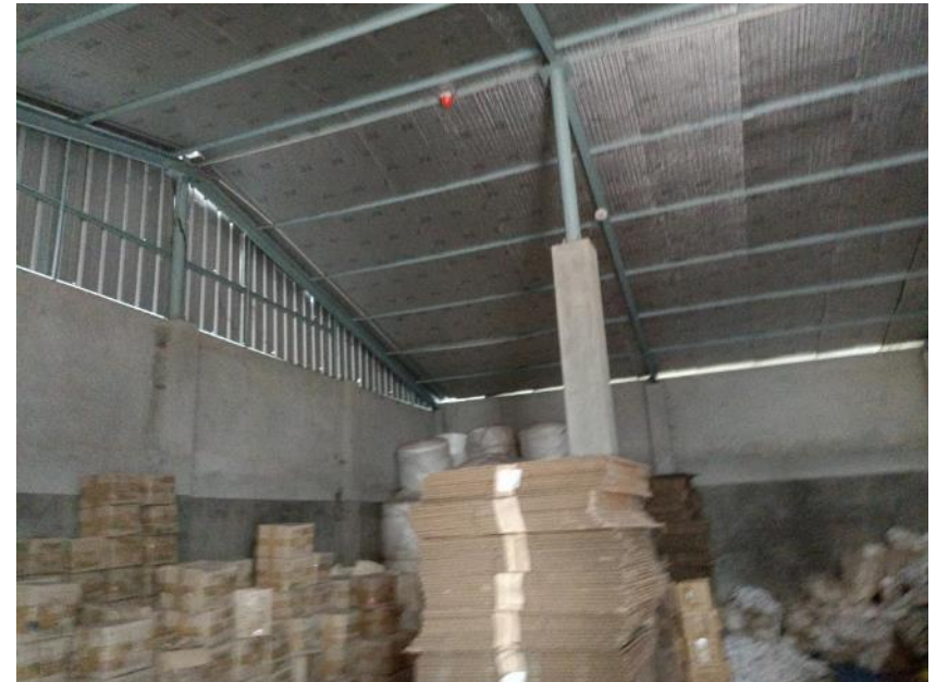
Load transfer media is missing at along long direction
