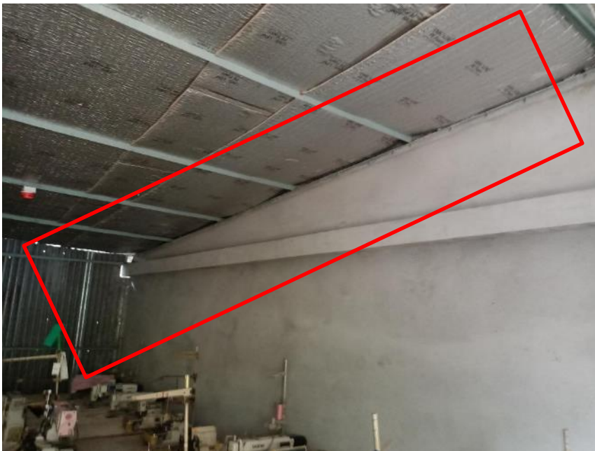
Apparently inadequate connection
