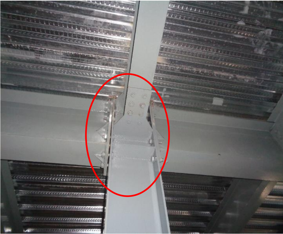
Gap was observed in connection
