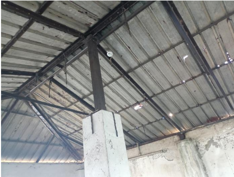
Roof shed of ETP Building
