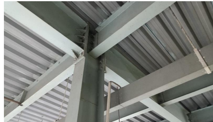
Sub beam & column connection
