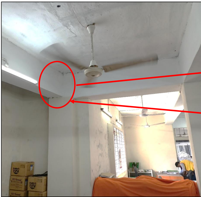
Crack found in Beam-Column Joint
