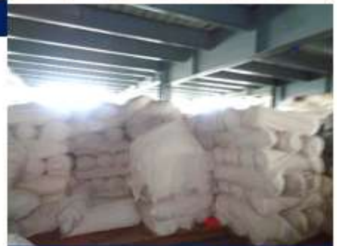
Yarn store (2 nd Floor), Steel part
