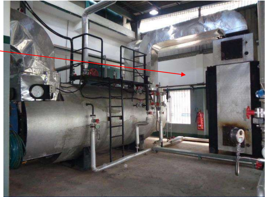
Onsite bracing condition
