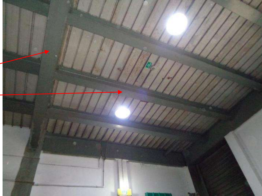
Onsite condition of 1 st floor steel beam
