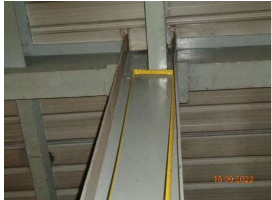
Onsite MB2 beam condition.
