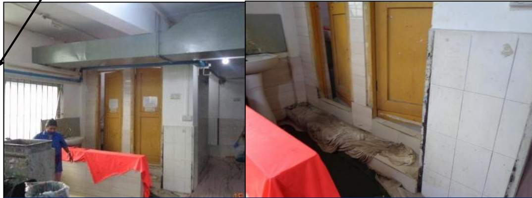
Additional room in front of stair
