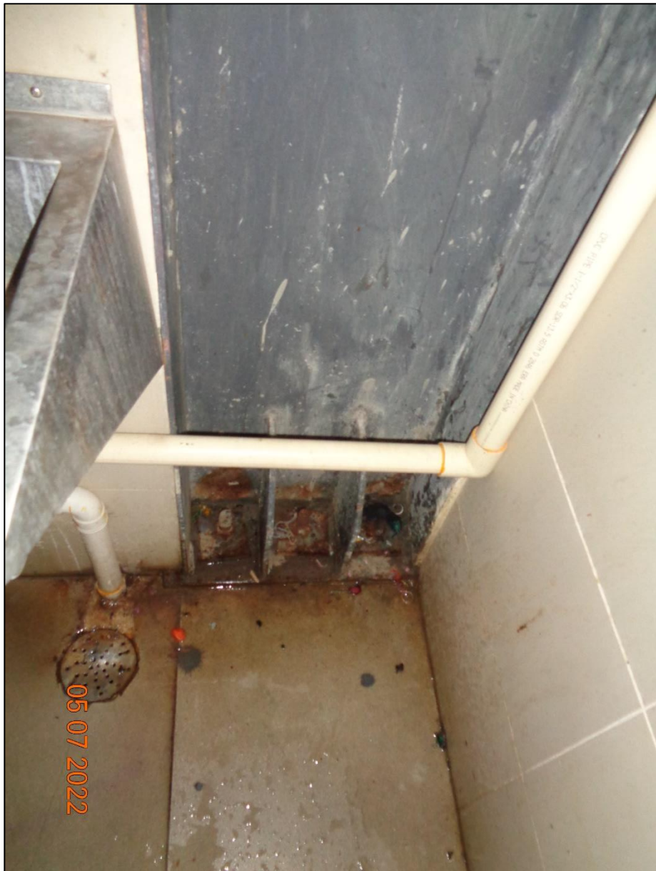
Corrosion in steel column
