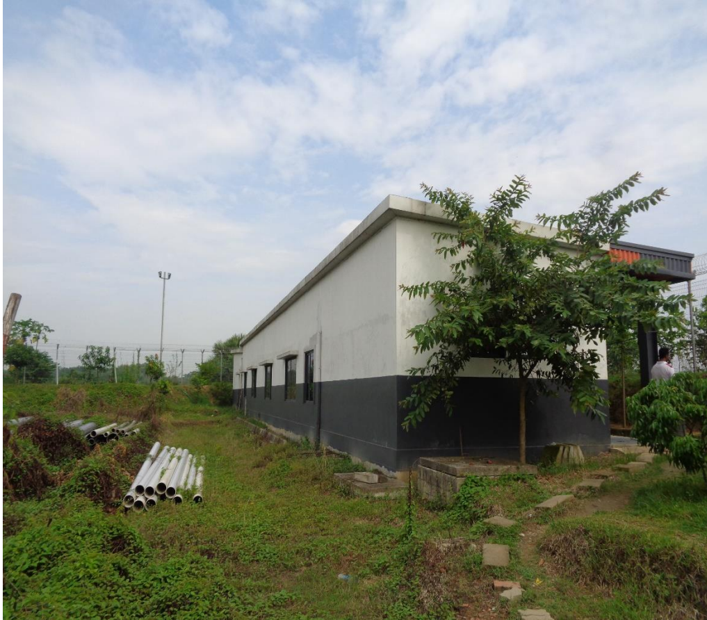
Security Dormitory Shed
