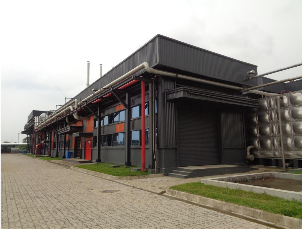
WTP & Pump House
