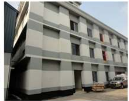
Building-06( 3-storeyed RCC)
