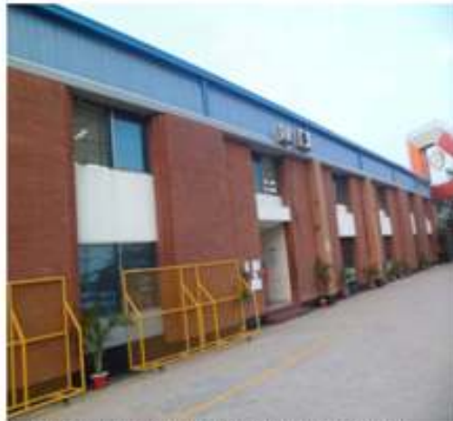
Building-02 ( 2-storeyed steel Build.)
