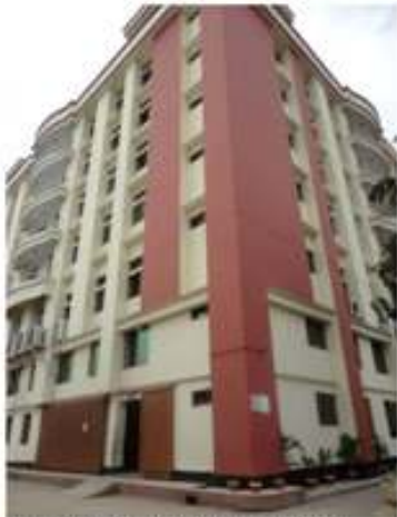
Building-01 (6-Storeyed RCC)
