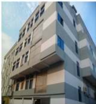
Building-04( 5-storeyed RCC)
