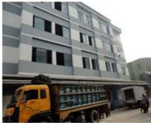
Building-05( 4-storeyed RCC)
