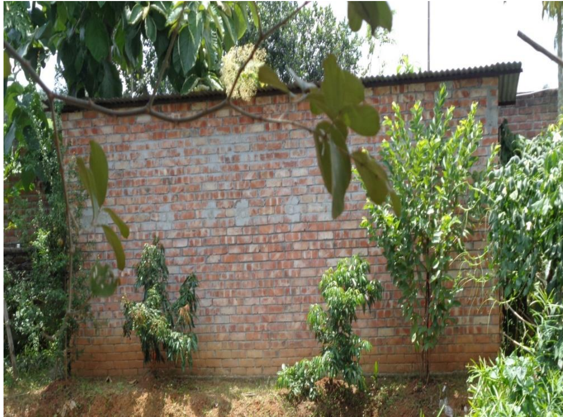
Building 6: Wastage Room
