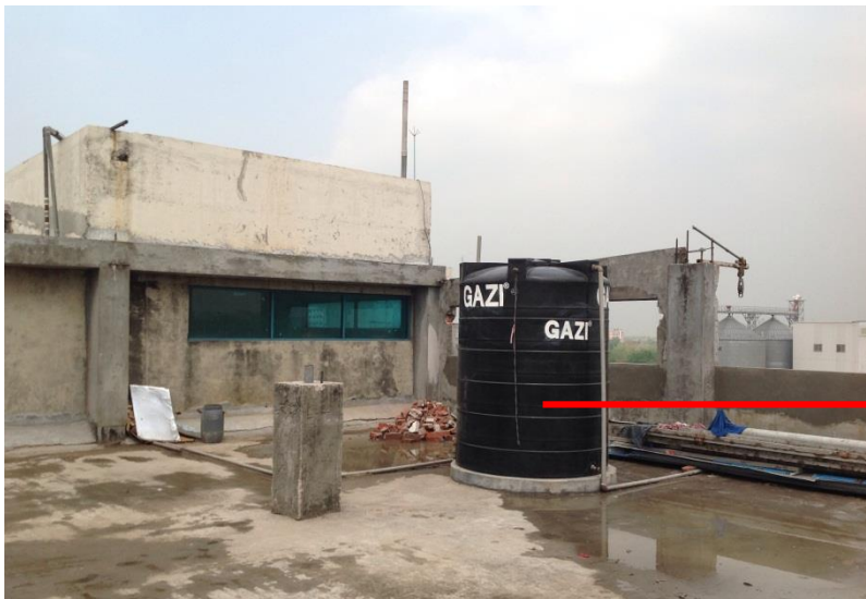
Roof - Plastic Water Tank
