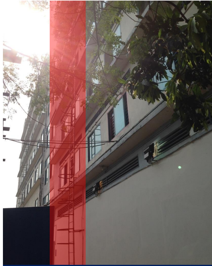
Fire escape ladder to West elevation
