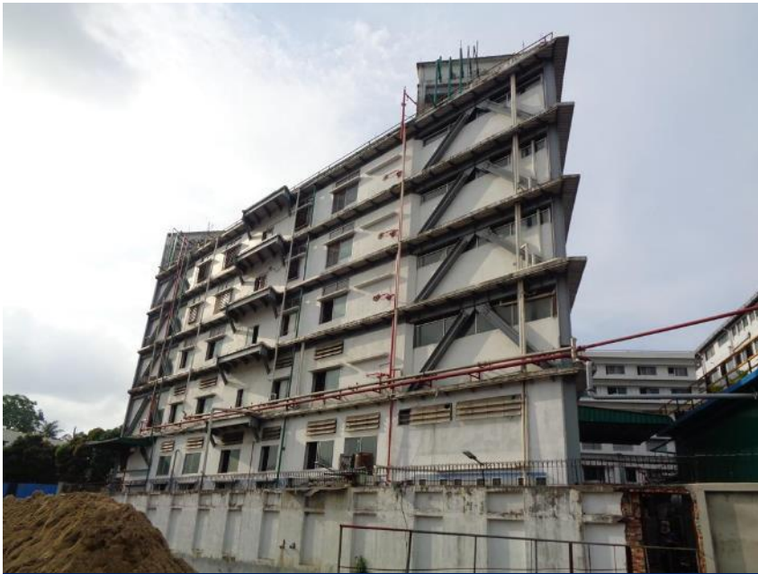
Vertical bracing (I-section)
