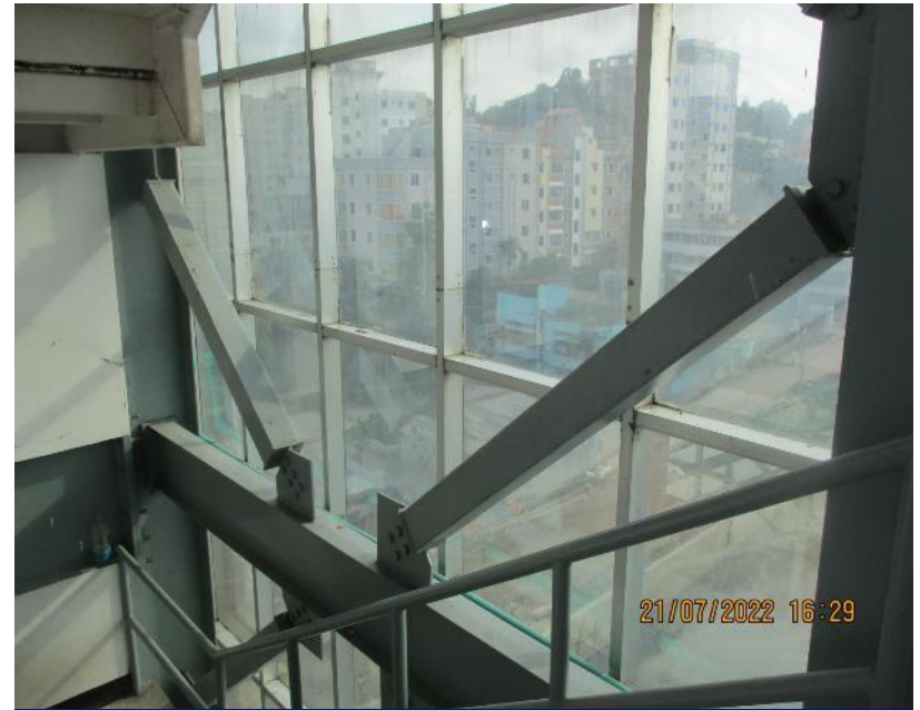
Vertical bracing (Box-section)
