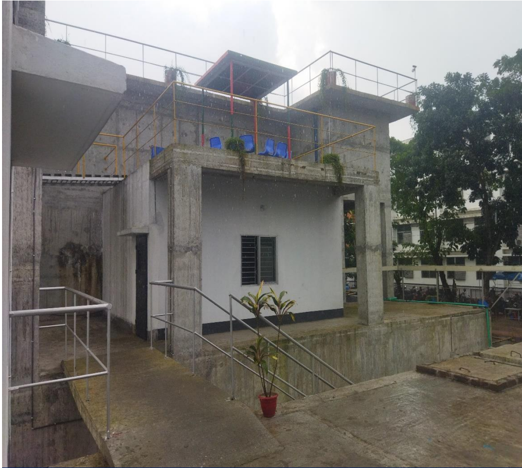
Building-10 (ETP & WTP)
