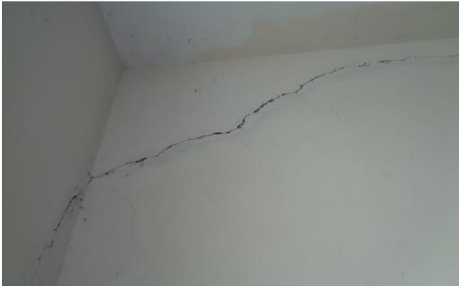
Crack in brick walls
