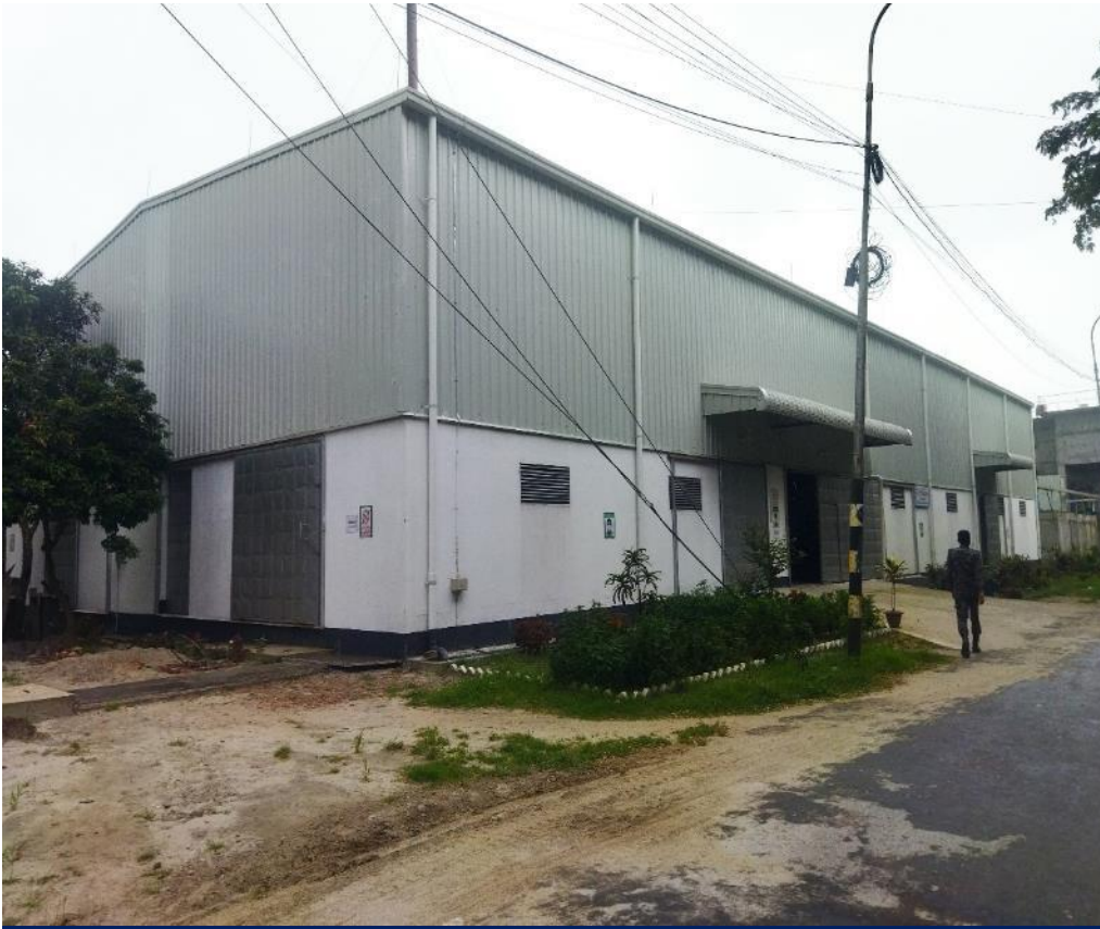
Building-9 (Utility Shed-2)
