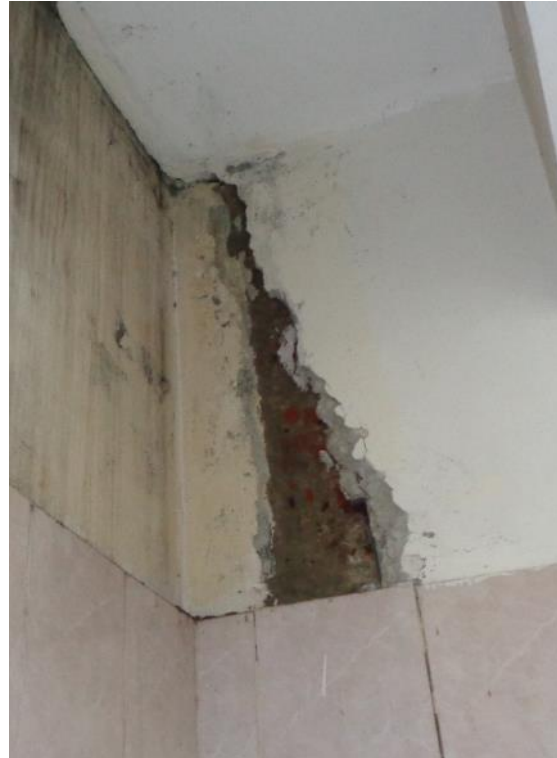
Crack in brick walls
