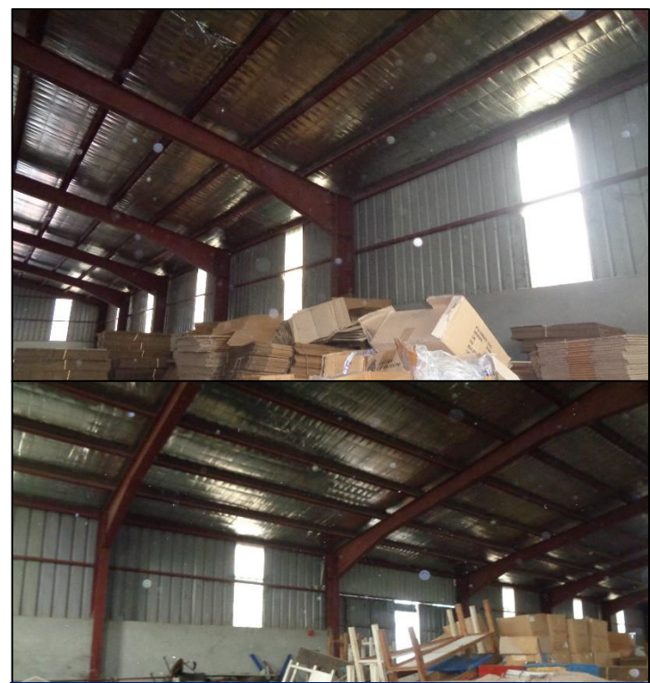
No load transfer media and bracing
