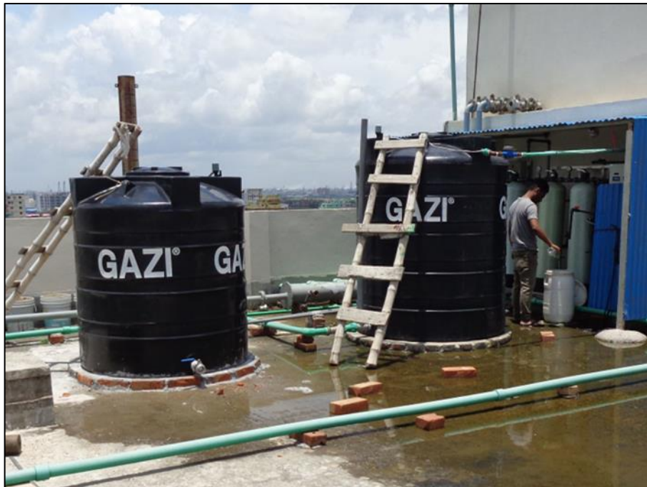
Plastic water tank on roof
