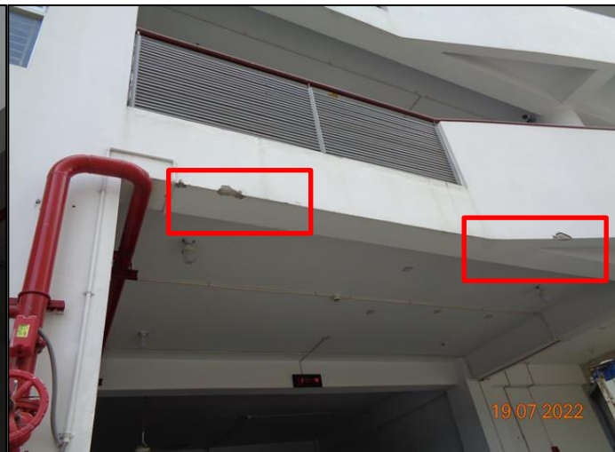
Beams are affected by the impact of vehicle
