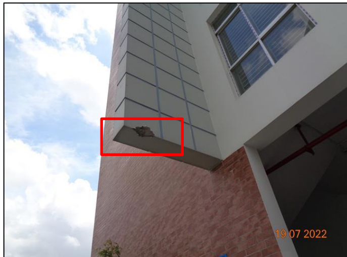
Beams are affected by the impact of vehicle
