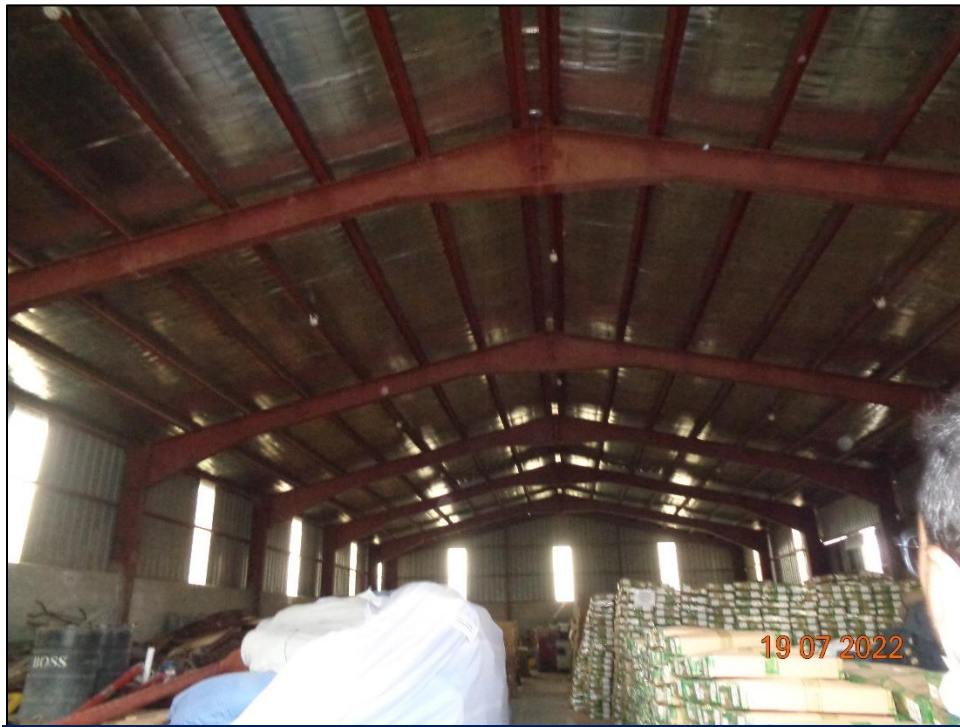
Steel portal frame
