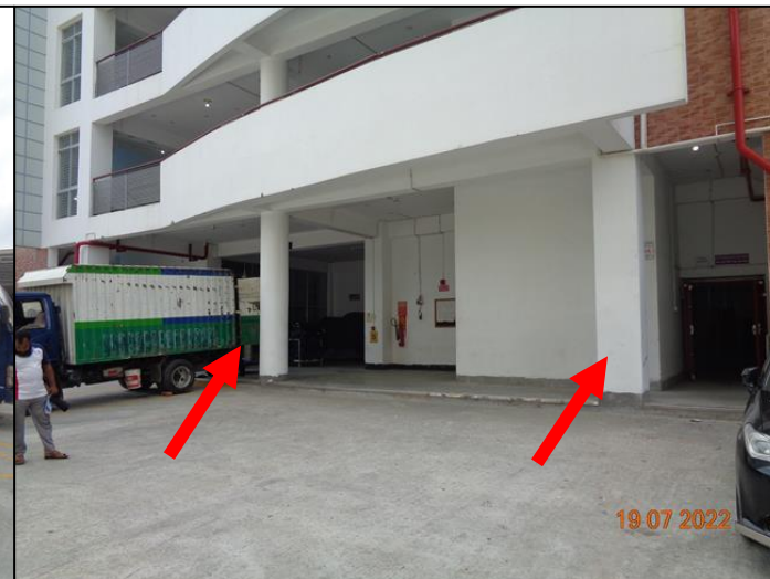
Columns having no barrier/protection at ground floor
