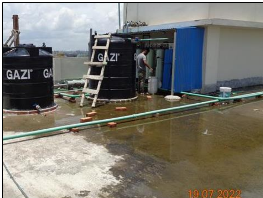
Water ponding at Roof
