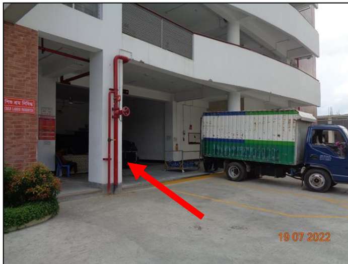
Columns having no barrier/protection at ground floor
