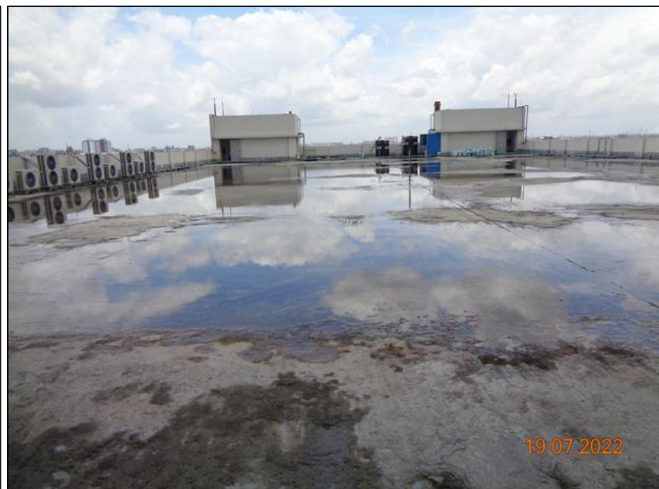
Water ponding at Roof
