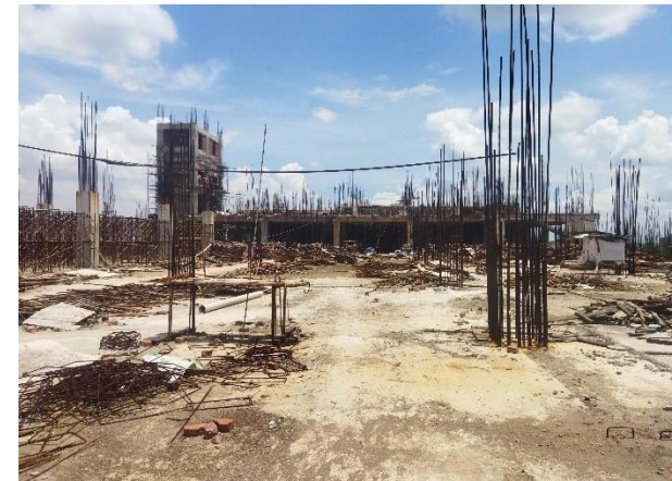
Ongoing extension work
