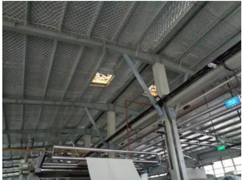
Lack of bracing at roof
