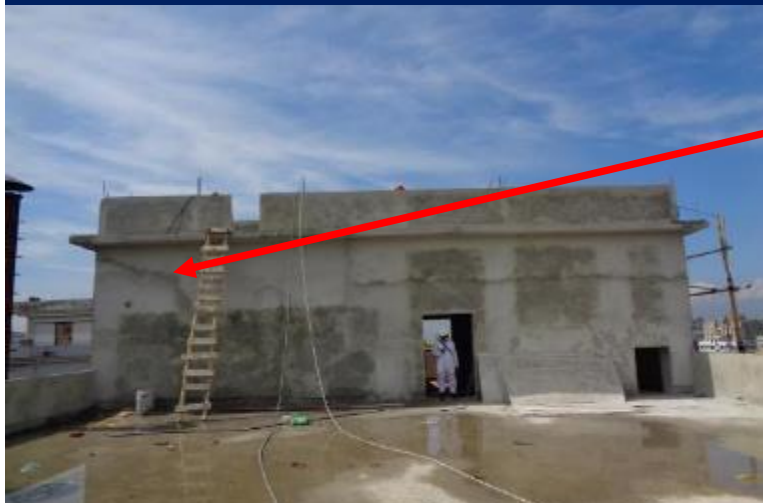
OHWT constructed over South East Staircase
