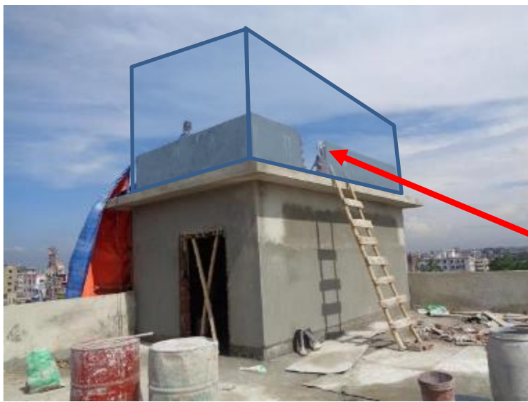
South East Staircase (OHWT not constructed)
