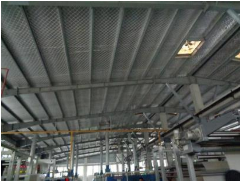
Lack of bracing at roof
