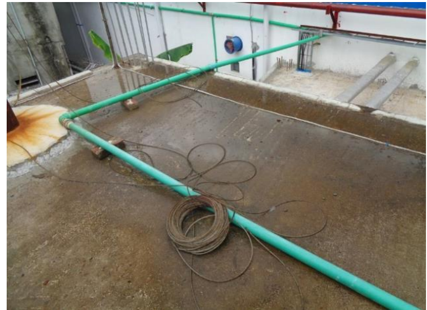
Standing water on the roof
