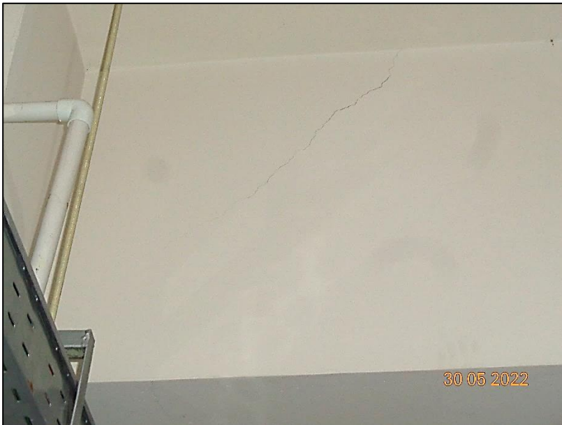
Cracks in several beam on 4 th floor
