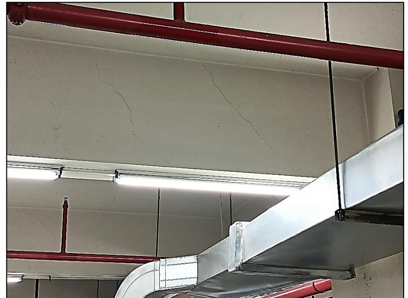
Cracks in several beam on 4 th floor
