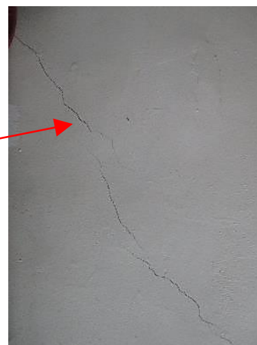
Crack on ground floor brick walls of north-east stair
