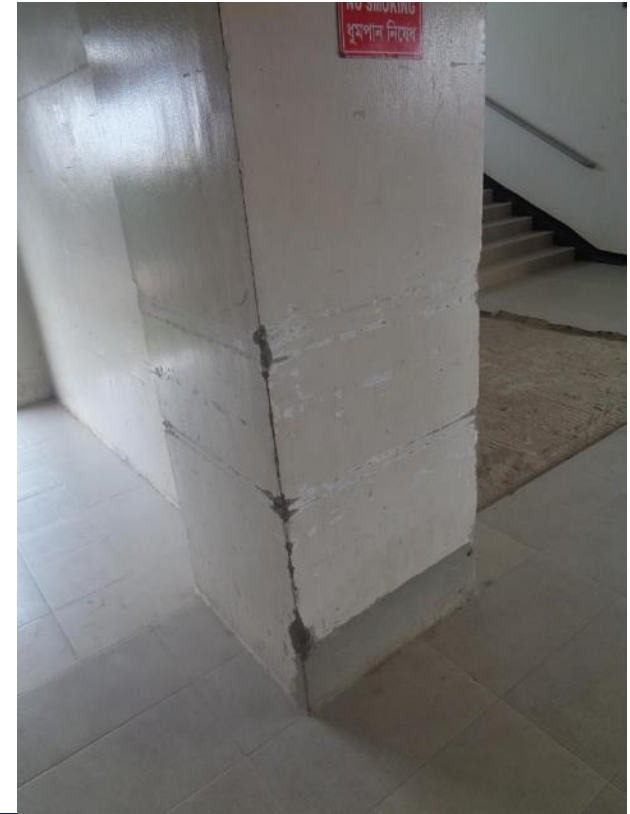
Damage of wall & column surface due to trolley impact
