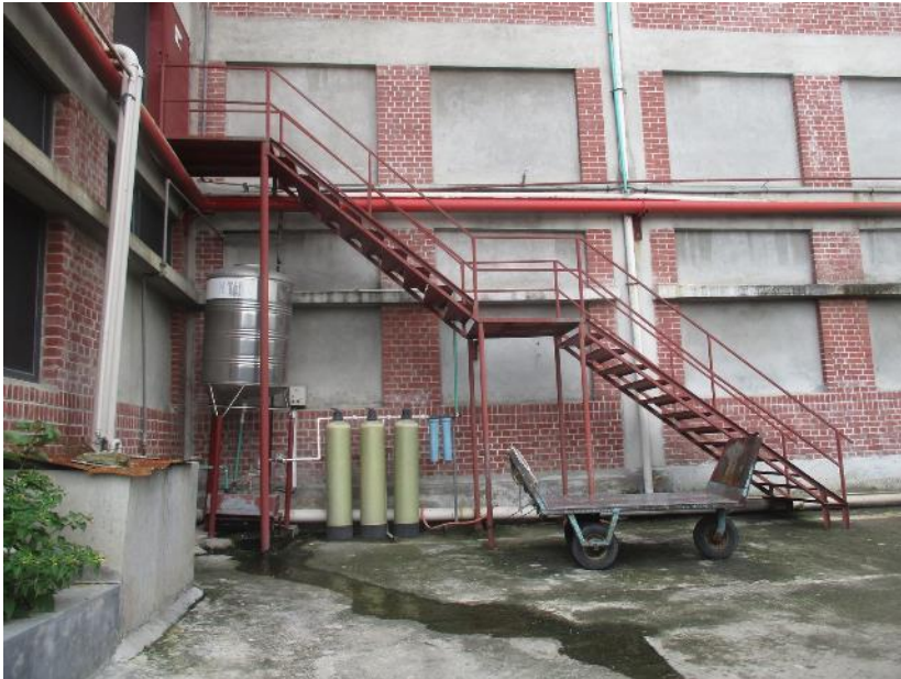
External steel stair adjacent to the Building-7
