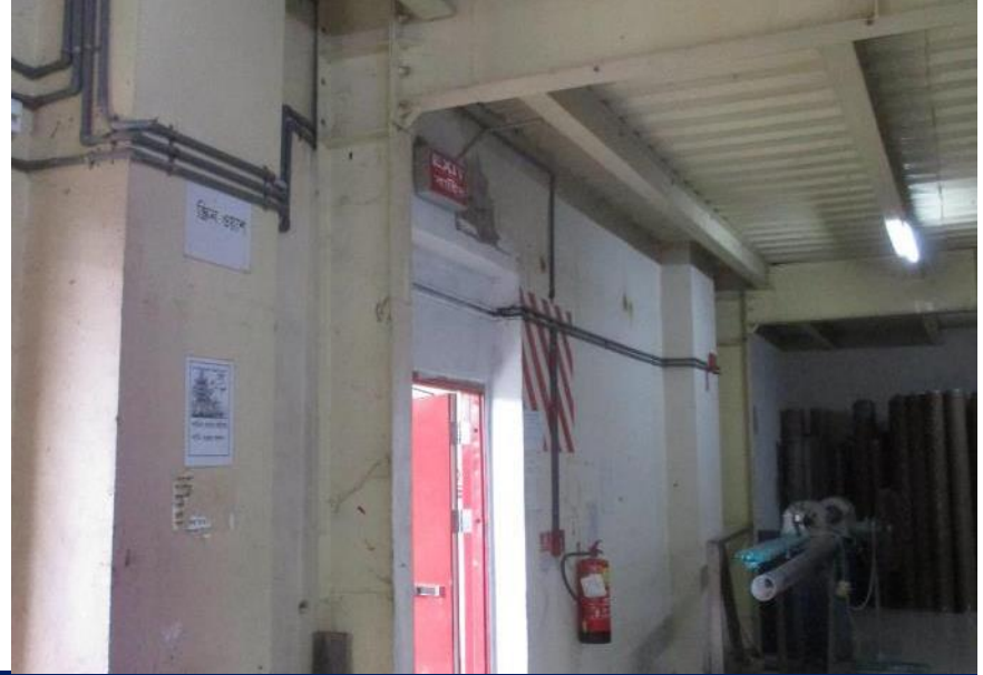
Portal frame without lateral bracing along long direction.
