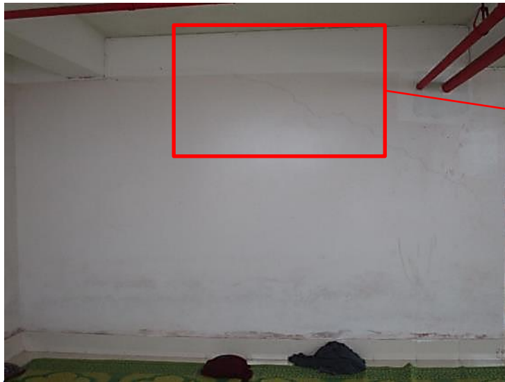
Crack on top floor brick walls of north-west stair
