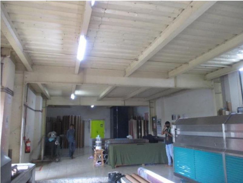
Portal frame without lateral bracing along long direction.
