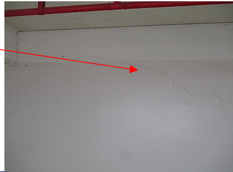
Crack on top floor brick walls of north-west stair
