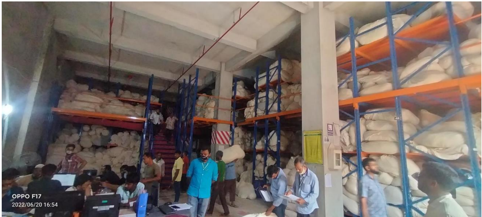
Steel storage rack and floor loading
