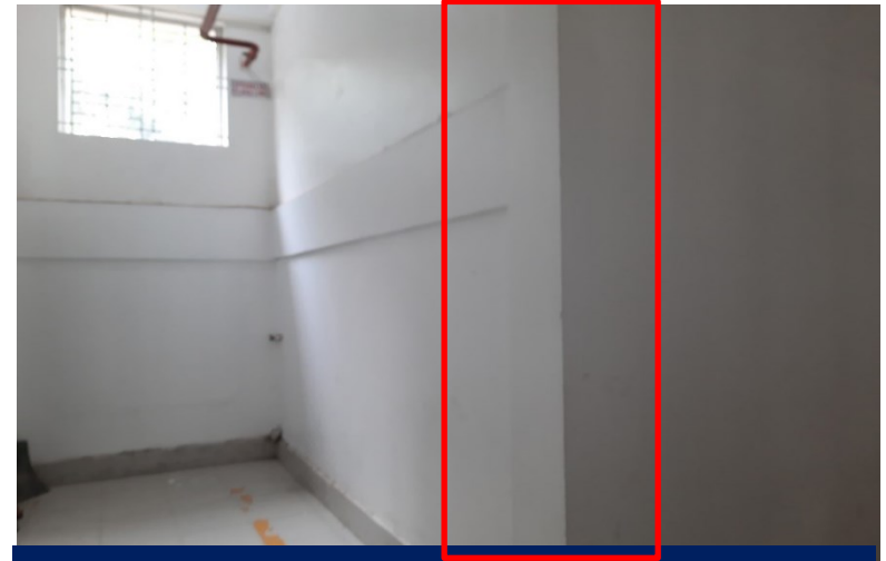
RC column in stair-2 (250 mm X 250 mm)
