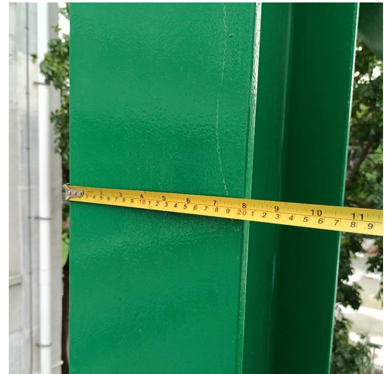
Flange width of steel column 200 mm
