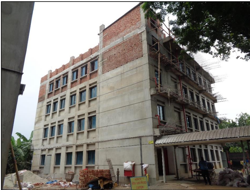
Existing 4 storied building
