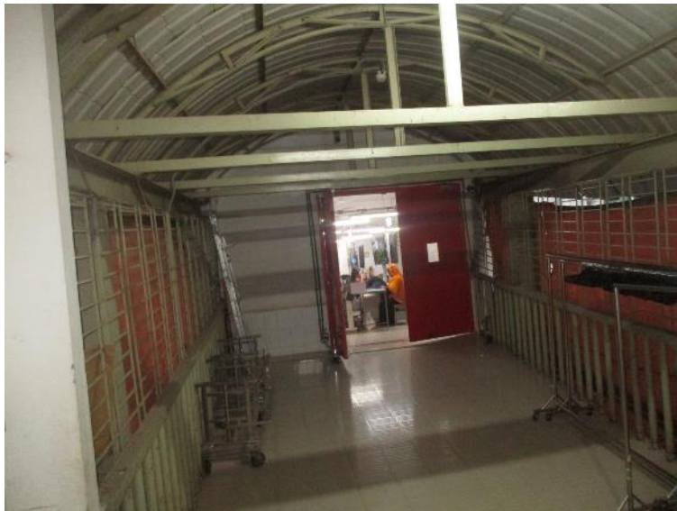
Steel Connecting Bridge
