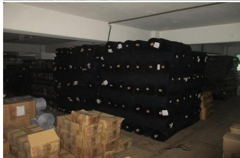
More than 4 kN/m 2 loading on steel racks
