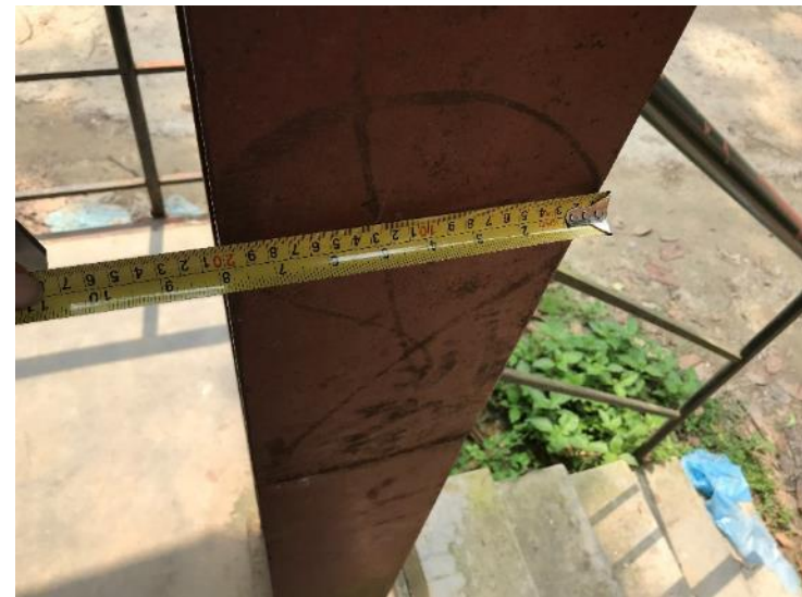
Steel Column Size- (W: 200 mmx 6 mm; F: 200 mm x 8 mm)
