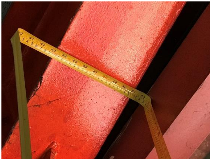
Steel Rafter Size- (W: 390 mm x 5 mm; F: 200 mm x 8 mm)
