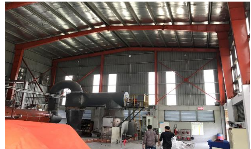
Angle bracing at end bays
