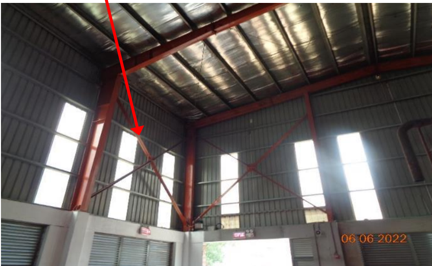
Tension/Angle bracing without compression strut
