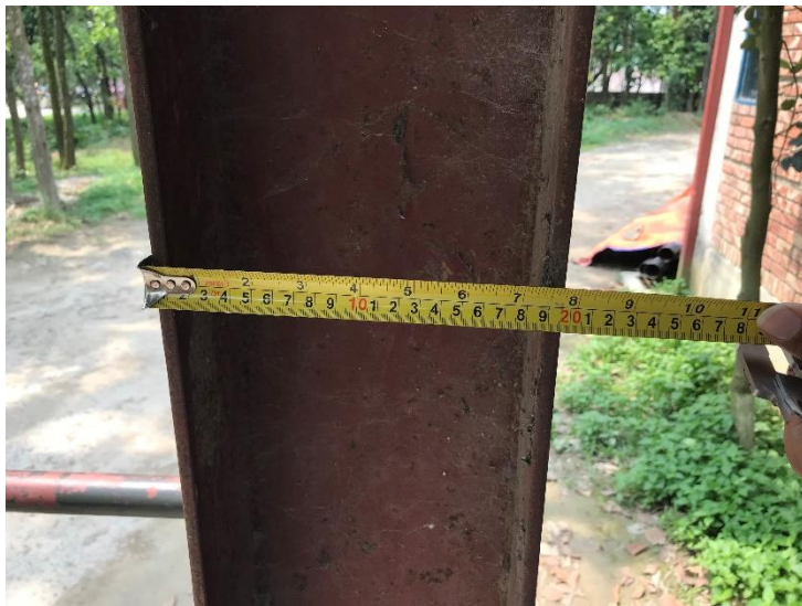
Steel Column Size- (W: 200 mmx 6 mm; F: 200 mm x 8 mm)
