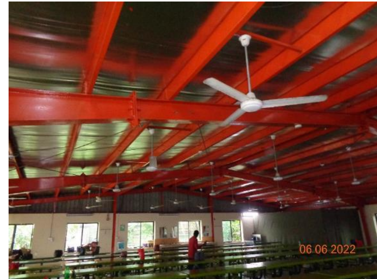
Lateral load transfer media missing at roof level
