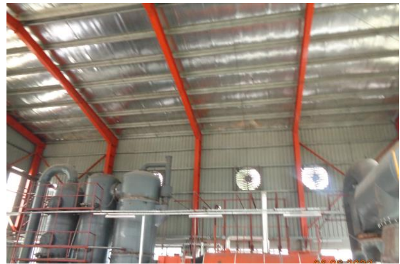
Lateral load transfer media missing at roof level
