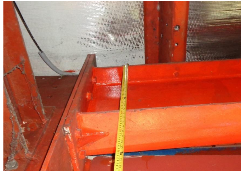
Steel Rafter Size- (W: 390 mm x 5 mm; F: 200 mm x 8 mm)
