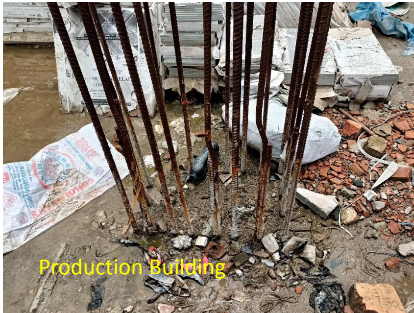
Exposed rebar at column on roof of Production & Warehouse Building
