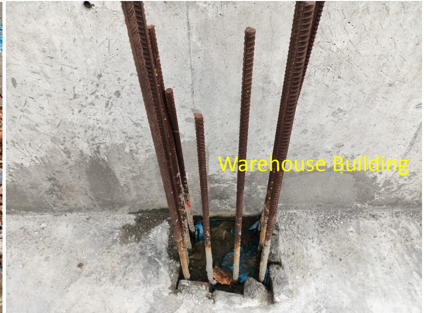
Exposed rebar at column on roof of Production & Warehouse Building
