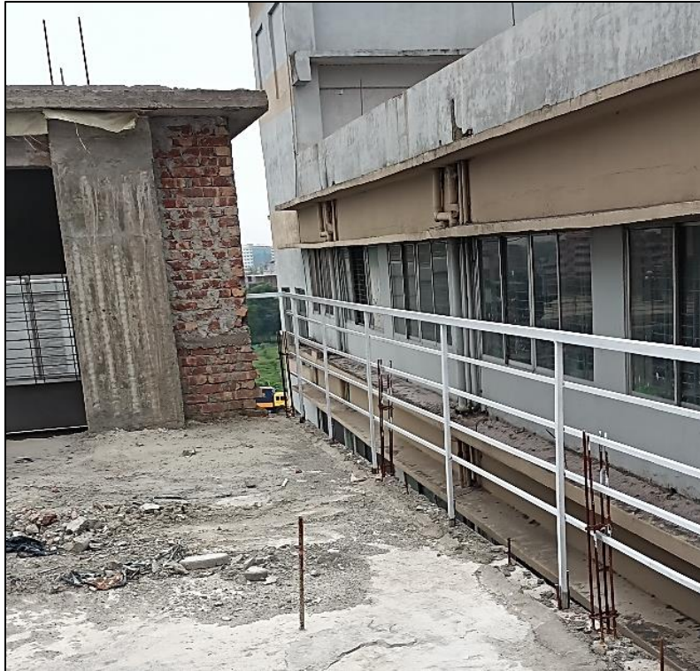
Exposed rebar at column on the roof
