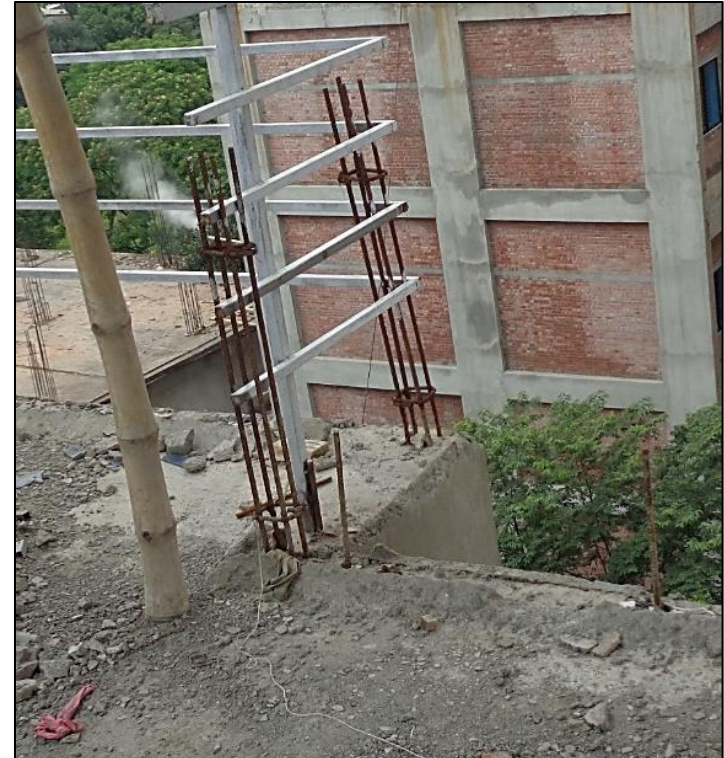
Exposed rebar at column on the roof
