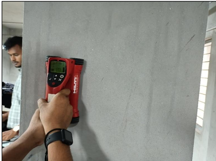
Rebar Scan by ferro-scanning
