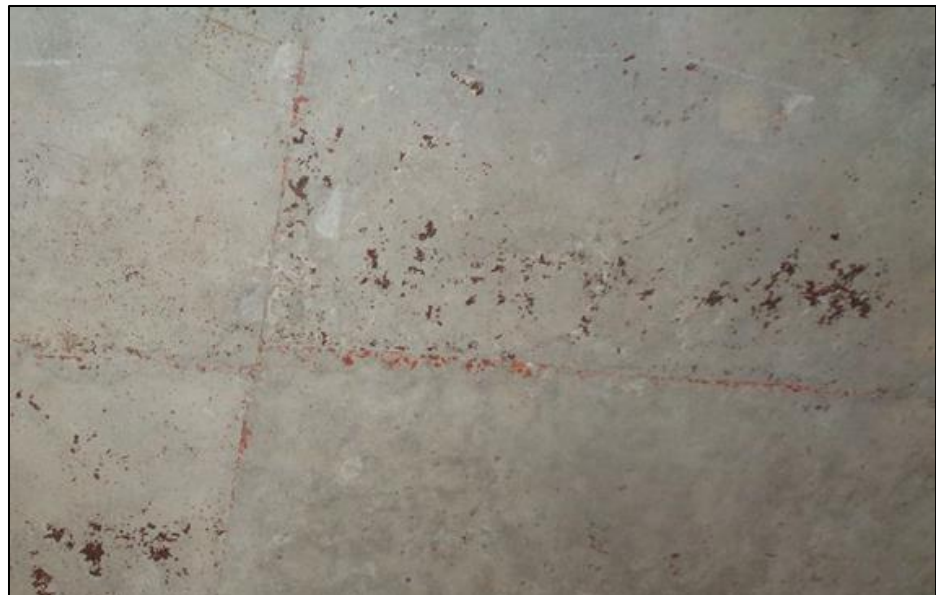
Brick Chips (Slab)c
