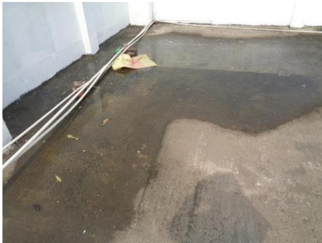
Standing water on the roof
