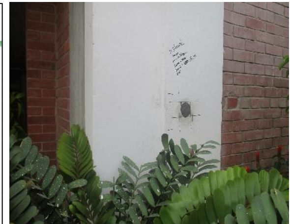
Concrete core observed at the column of Facility Building
