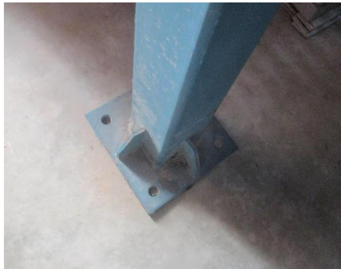
Storage rack not anchored or braced
