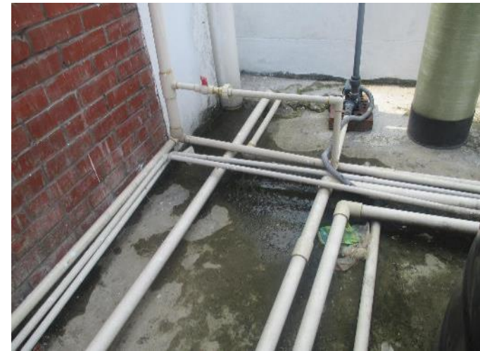
Standing water on the roof
