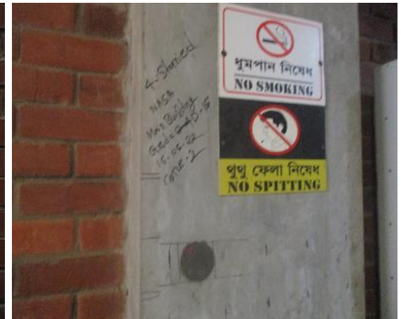
Concrete core observed at the column of Office Building
