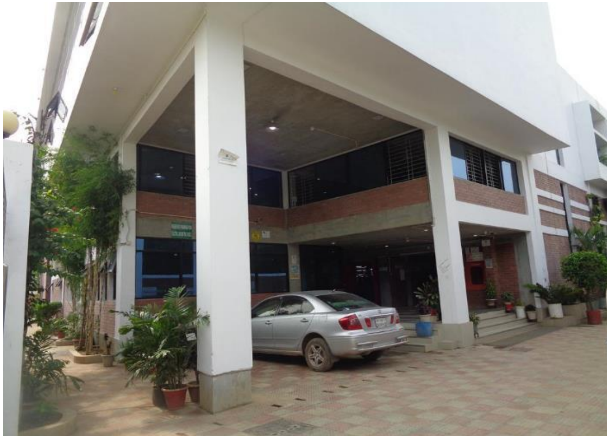
Ground Floor Column at Parking
