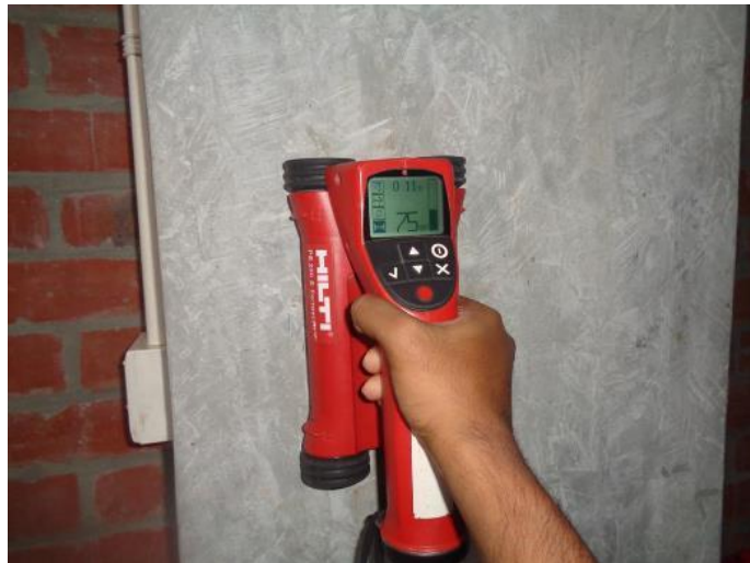
Rebar Scanning to verify rebar
