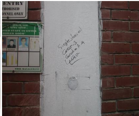
Concrete core observed at the column of Utility Building
