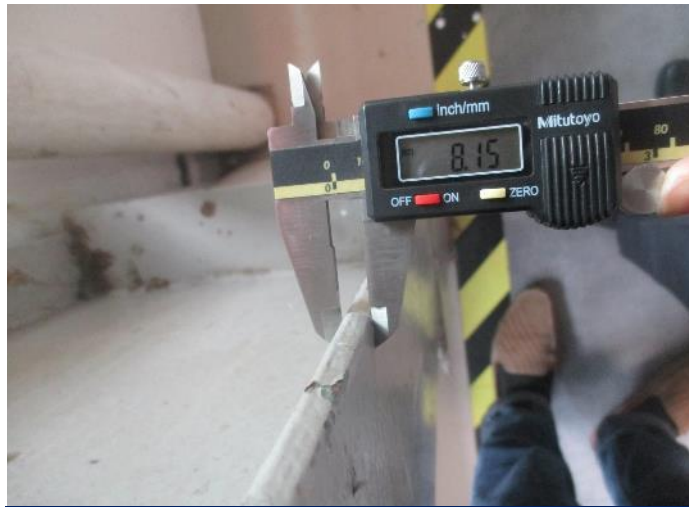
Steel Member Measurement
