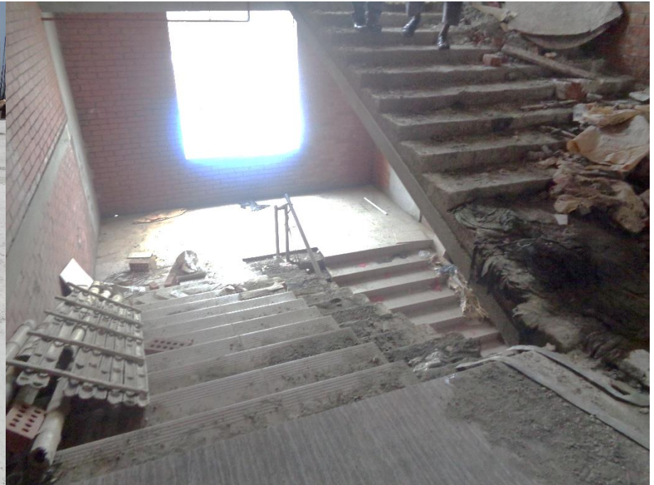
Parapet/railing was missing at roof and stair area
