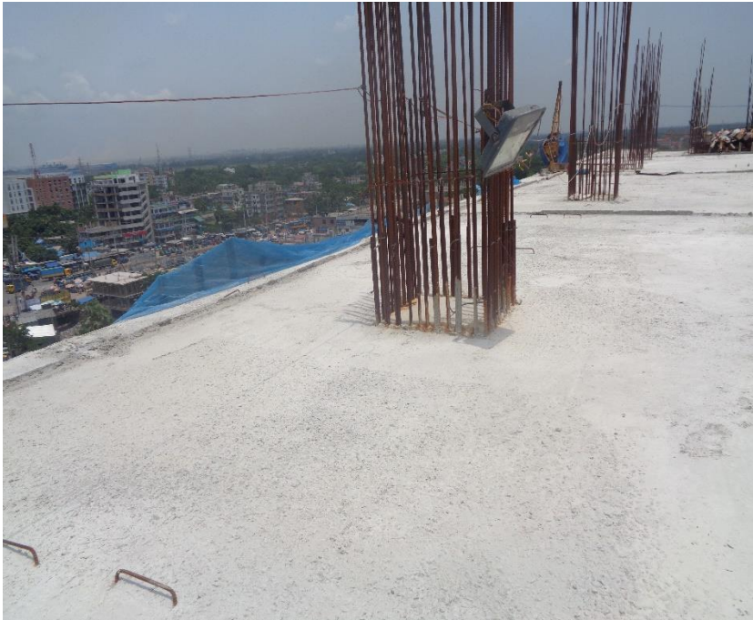
Parapet/railing was missing at roof and stair area
