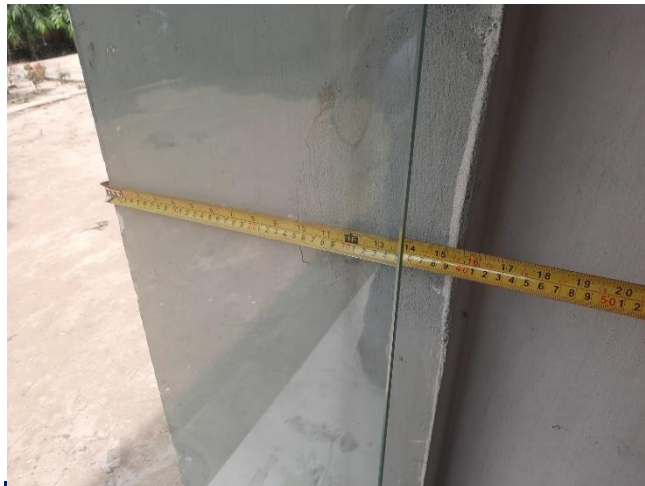
On site column size (375X500 mm)
