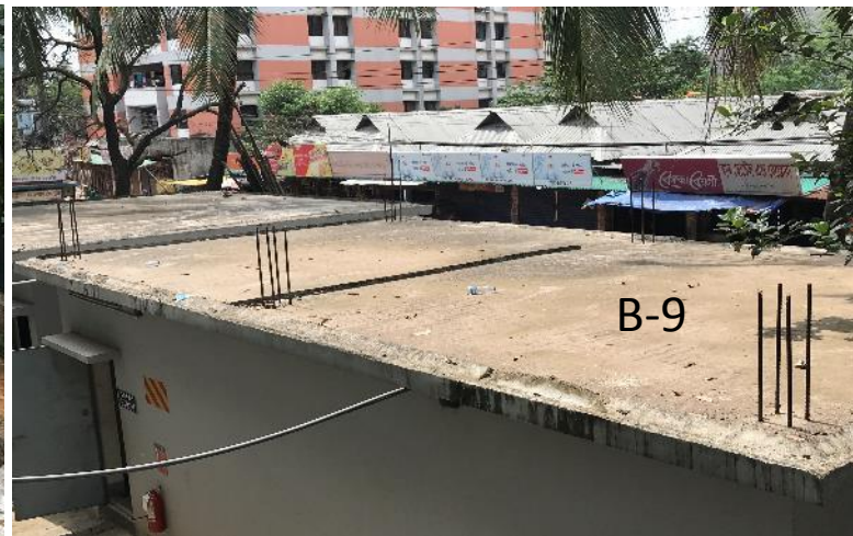
Corrosion on exposed rebar at roof
