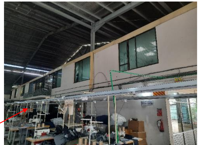
On site Mezzanine floor at north side
