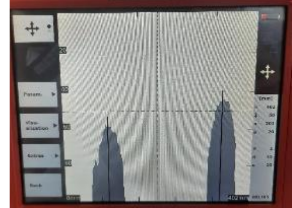
C1 column rebar by ferro scanning
