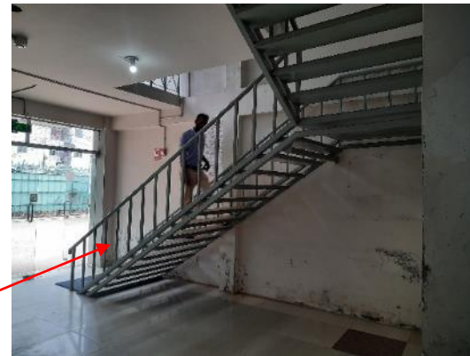
On site steel stair
