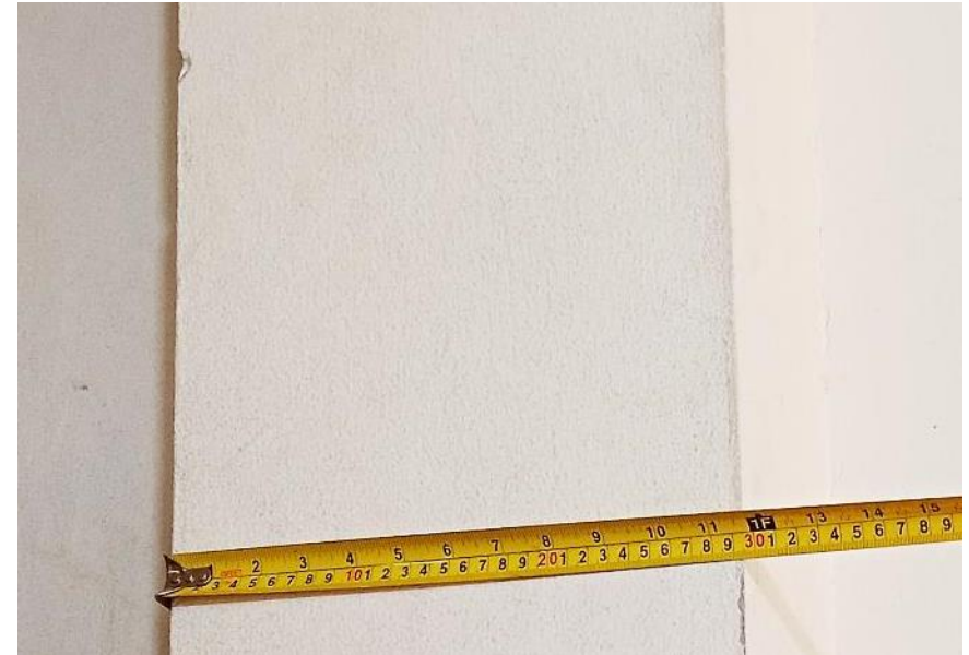
Existing column size (250X300 mm)
