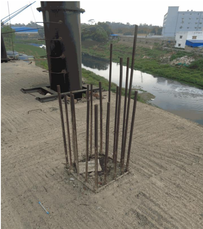
Corroded exposed rebar at roof
