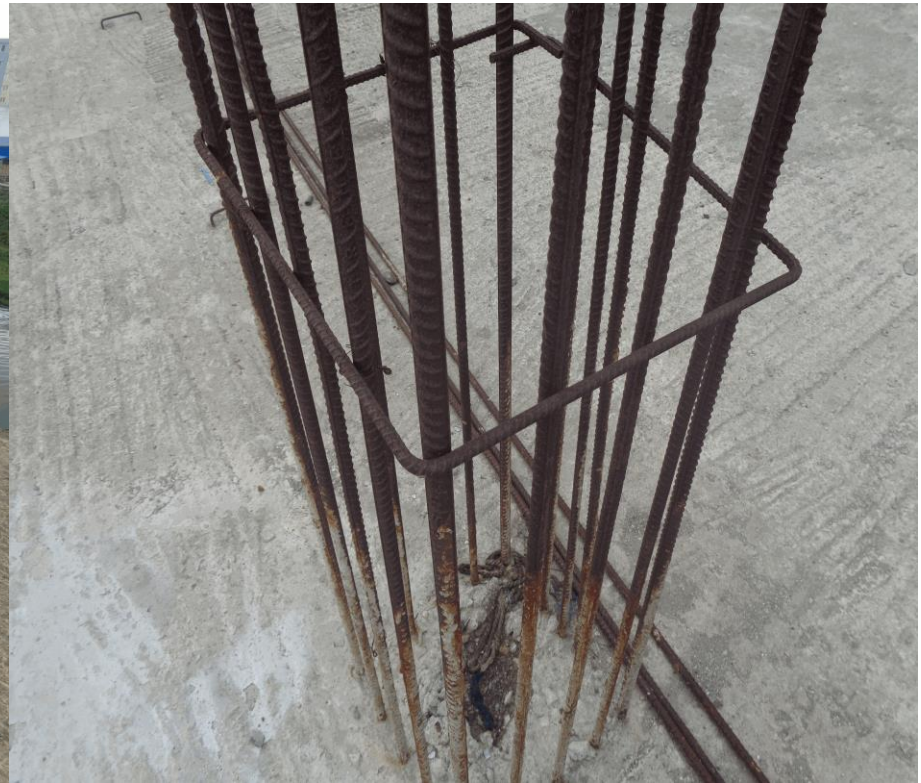
Corroded exposed rebar at roof
