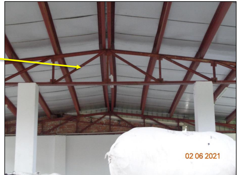
Orientation of truss diagonal members
