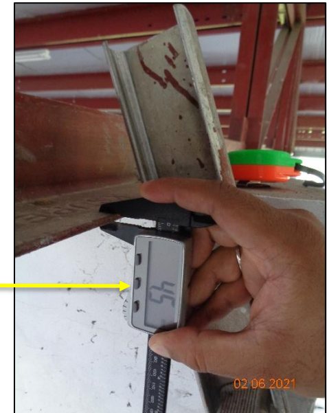
Measurement of truss bottom angle thickness
