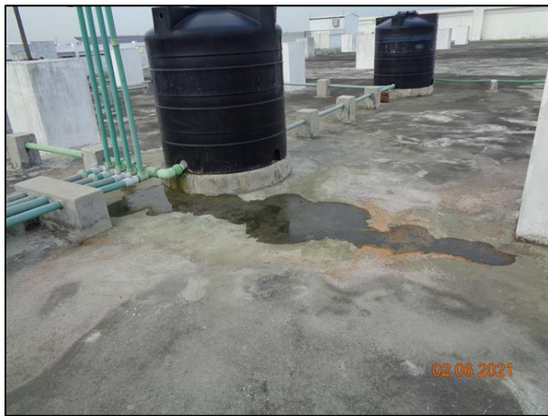
Leakage in water supply line
