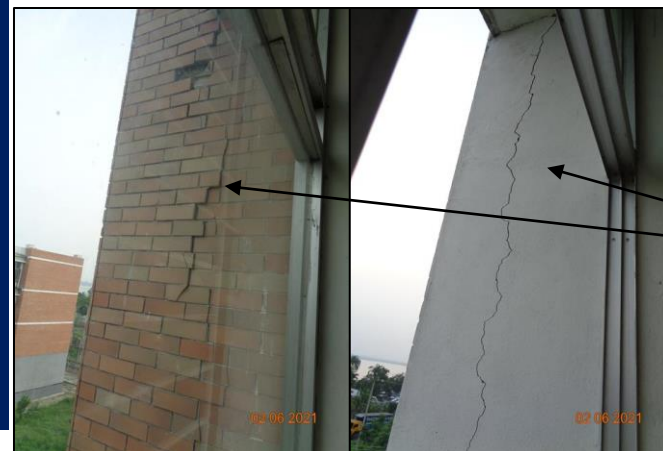
Crack in brick wall
