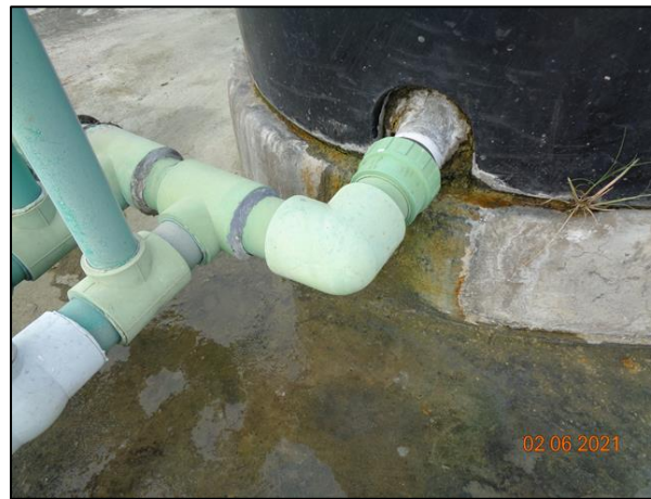
Leakage in water supply line
