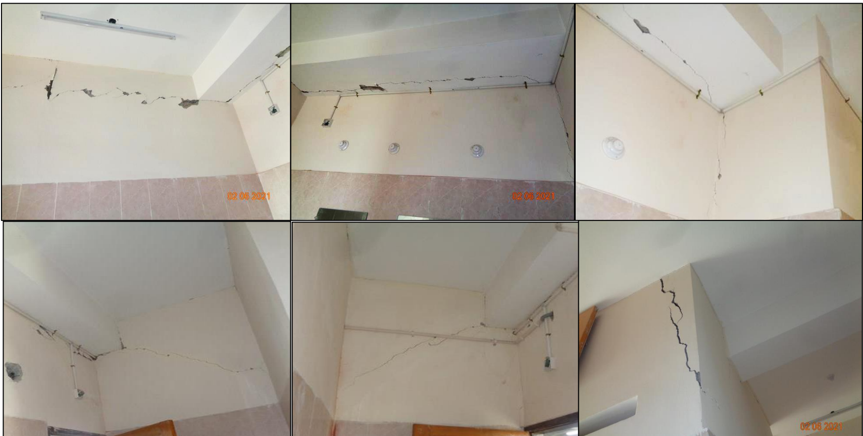
Crack in brick wall
