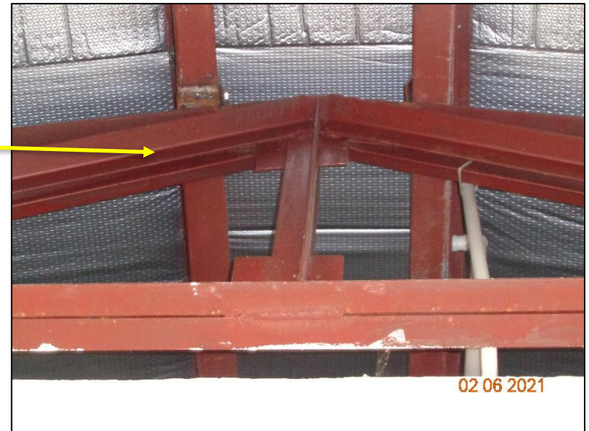
Orientation of truss diagonal members
