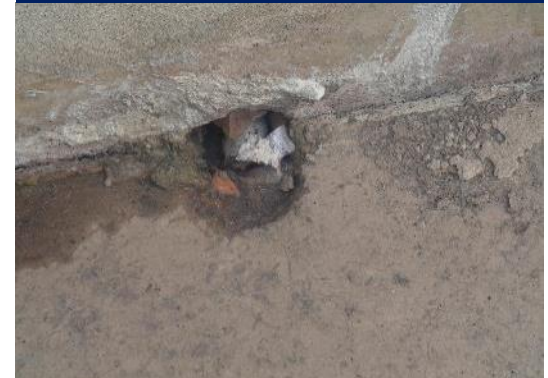
Inactive outlet at the roof of Building-2
