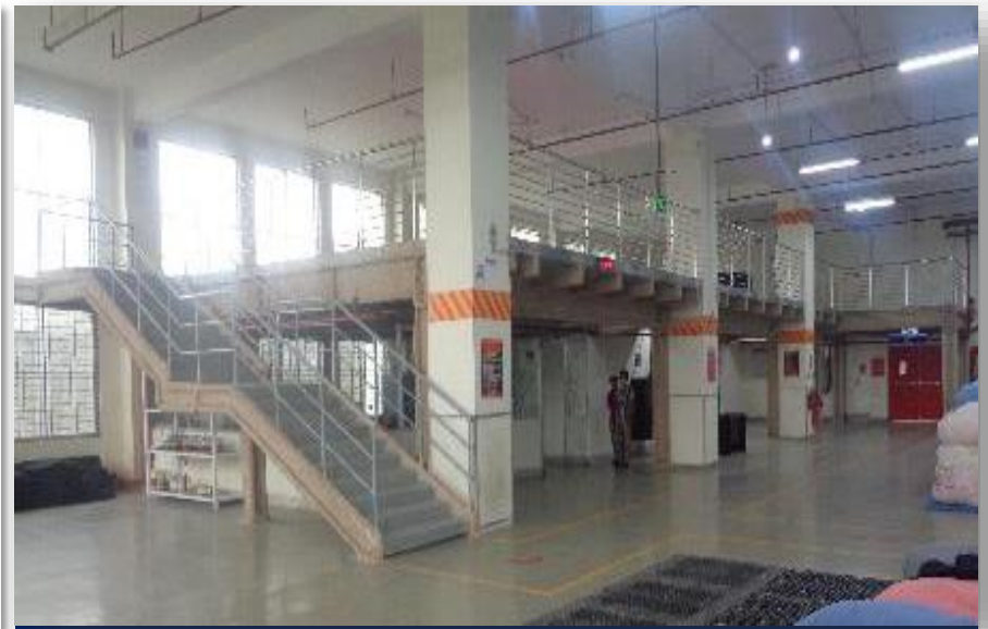
Self supported steel mezzanine floor
