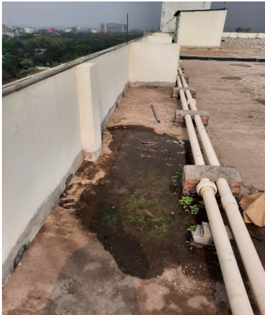
Water ponding at the roof of Building-1
