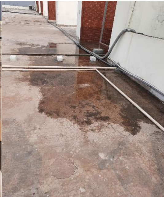
Water ponding at the roof of Building-1
