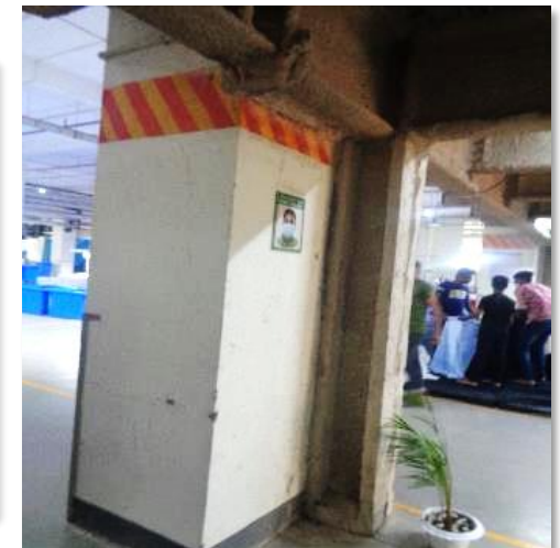
Steel mezzanine floor column on ground slab
