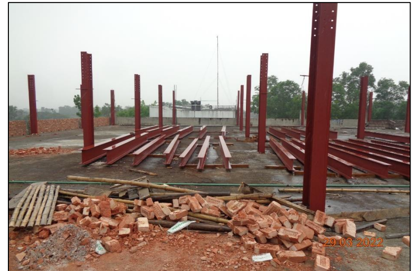
Ongoing construction on 2nd floor
