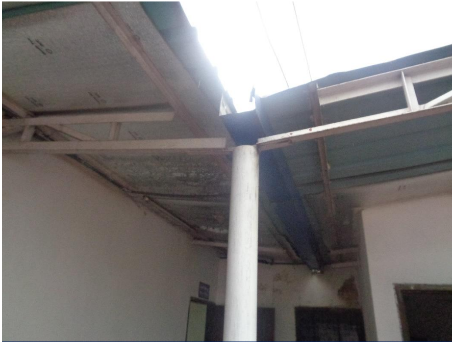
Connection of truss to steel pipe and brick wall
