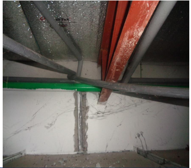
Connection of truss to steel pipe and brick wall
