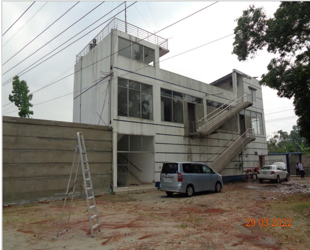
Office Building-front view
