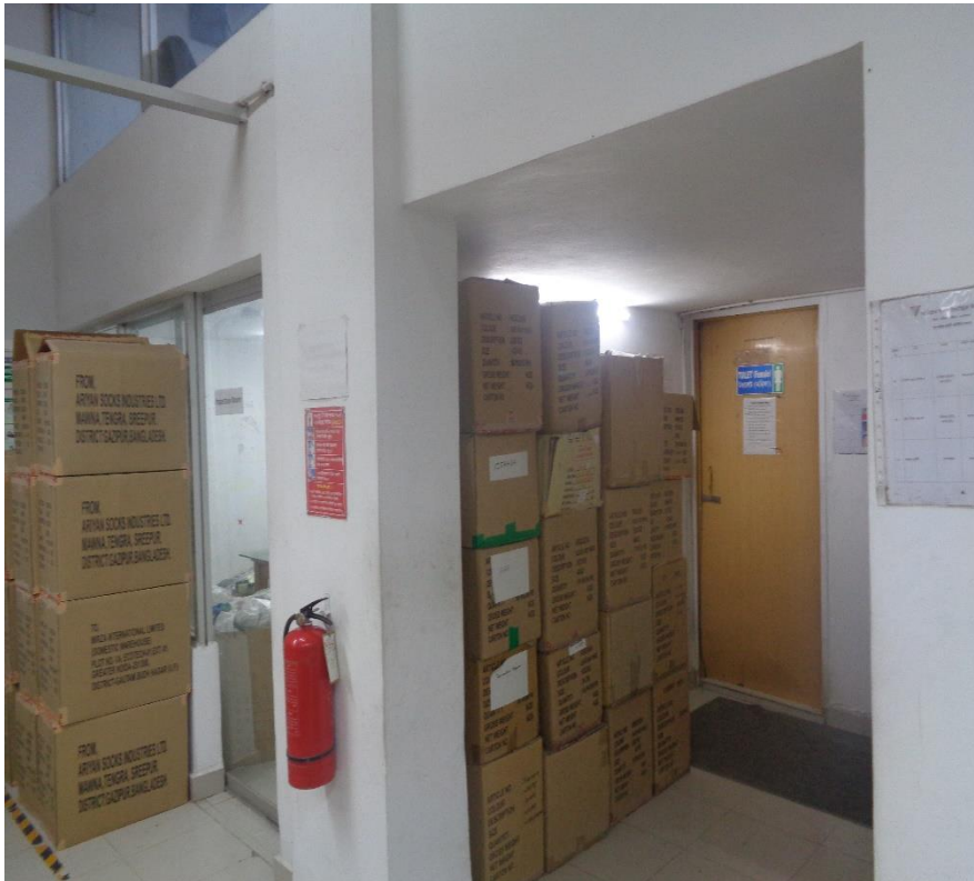
Dimension or thickness of mezzanine floor slab not shown in drawing
