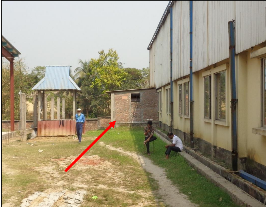
Toilet block at north-east corner
