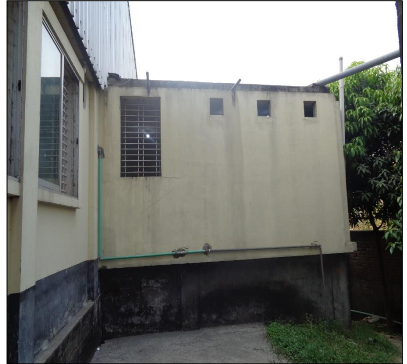
Toilet block at east side
