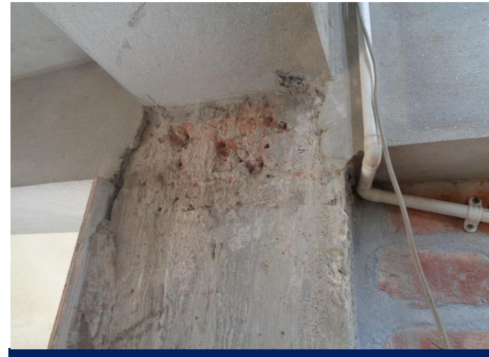
Security Building: Brick aggregate
