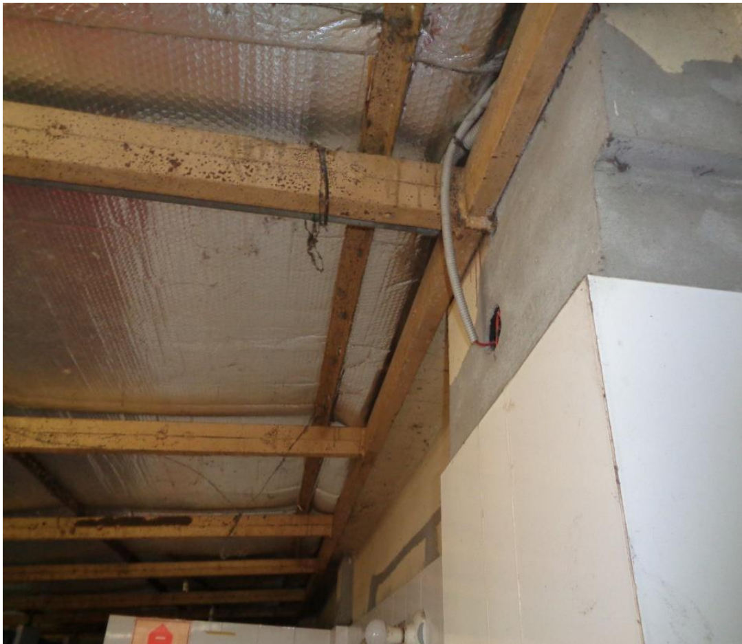
Toilet block at north-east corner
