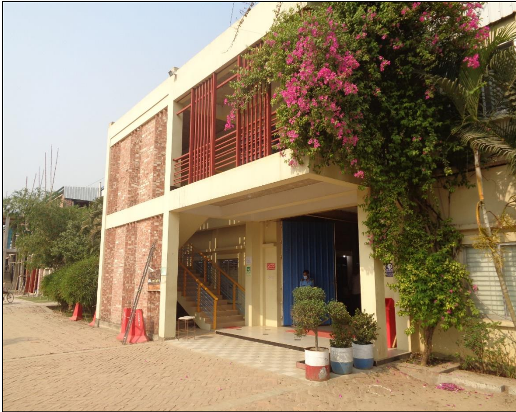
Independent RC Stair at Shed-1 (Factory Building)
