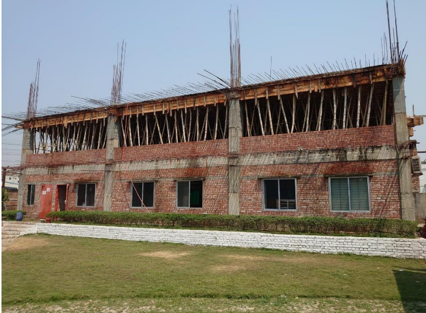
Exposed rebar of floors
