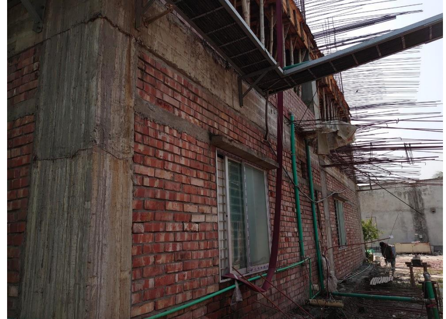
Exposed rebar of floors
