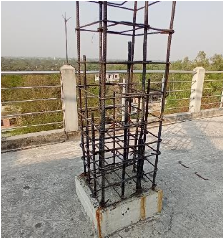
Corroded exposed rebar at roof
