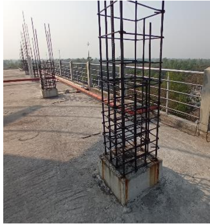
Corroded exposed rebar at roof
