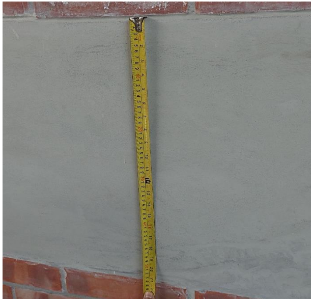
Existing beam dimension (300x 500)
