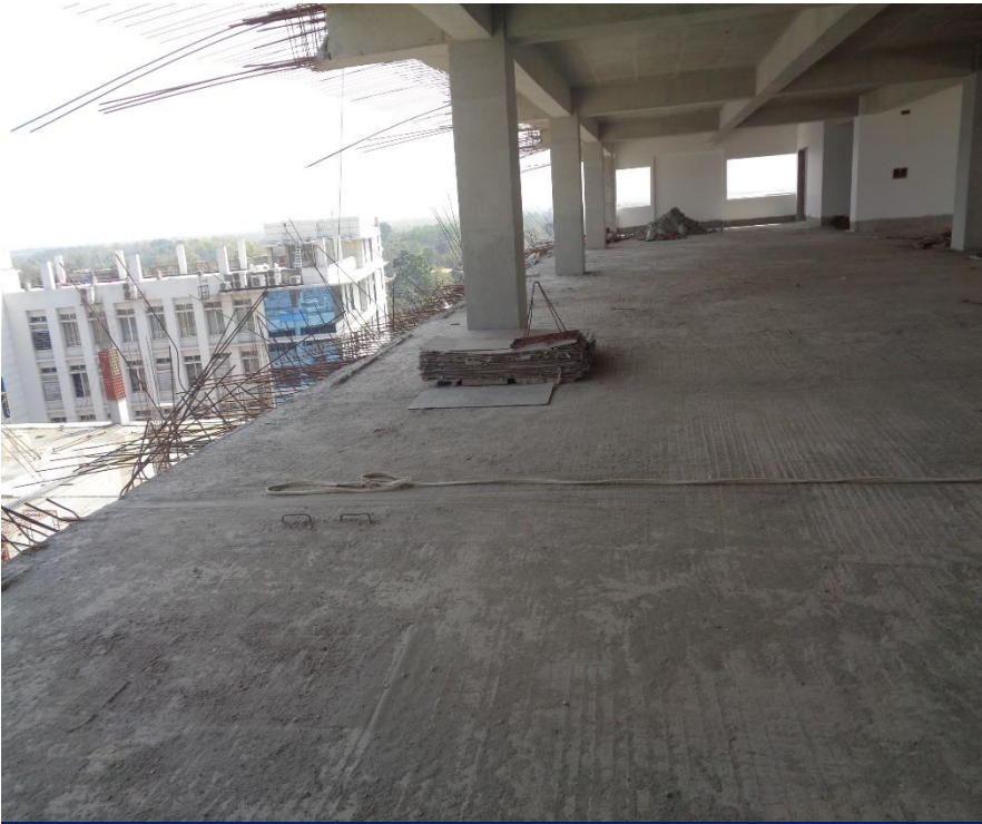
No edge protection provided at existing 6 th , 7 th floor and roof
