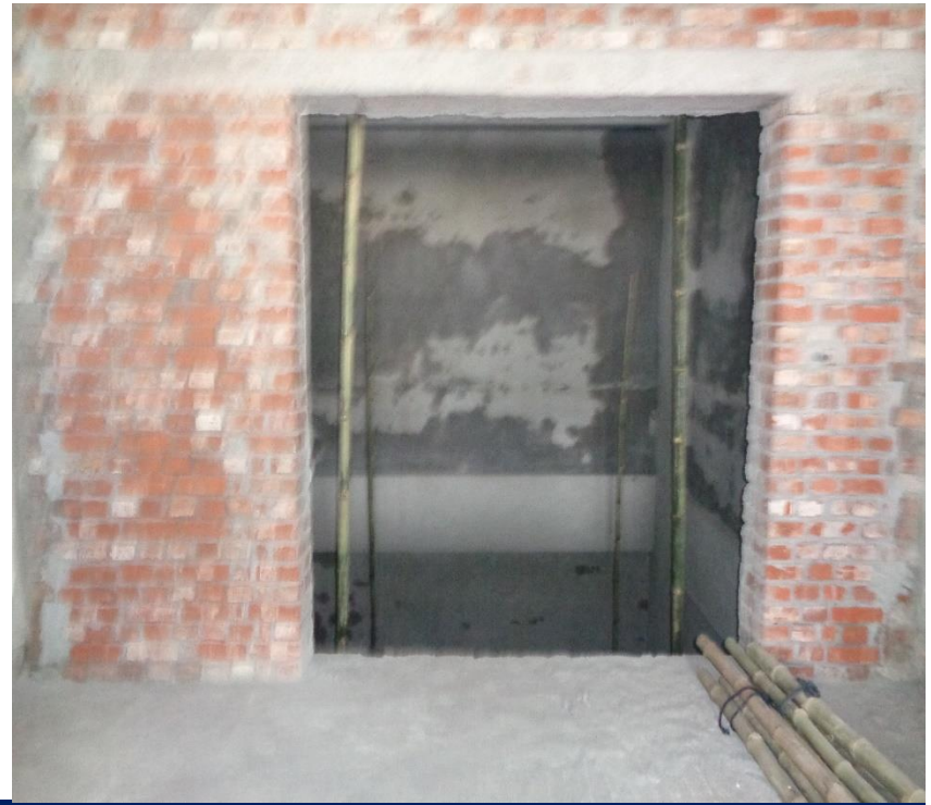
No edge protection provided at existing 6 th , 7 th floor and roof
