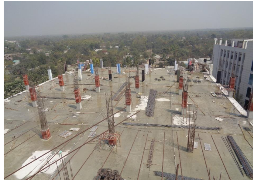
Ongoing construction on 5 th floor
