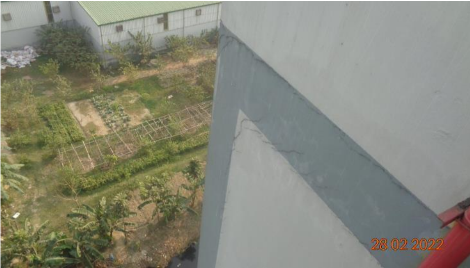
Fig- Crack on façade wall
