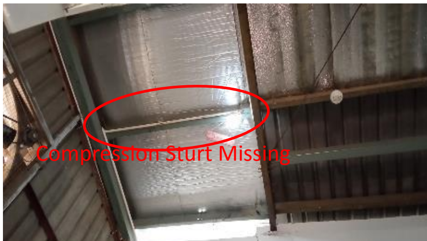
Compression Strut Missing
