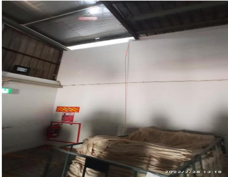
Crack on the brick wall
