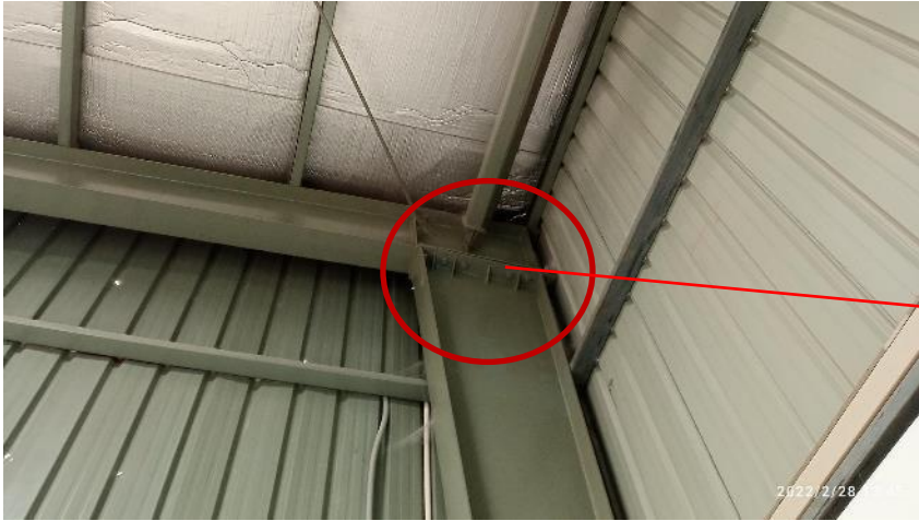
Gaps between connection plates
