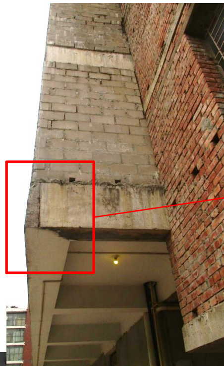
Crack in cantilever beam edge
