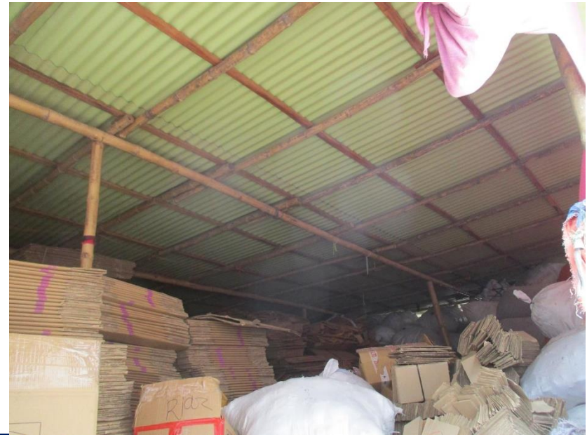
Undocumented temporary wastage shed made by bamboo frame.
