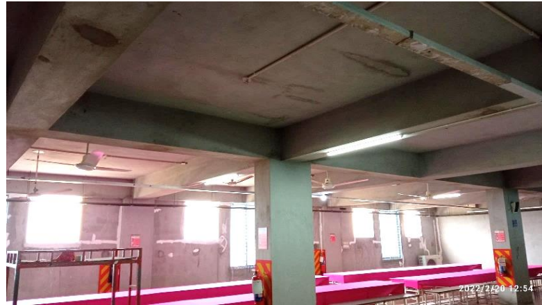
Sign of water ponding on roof slab
