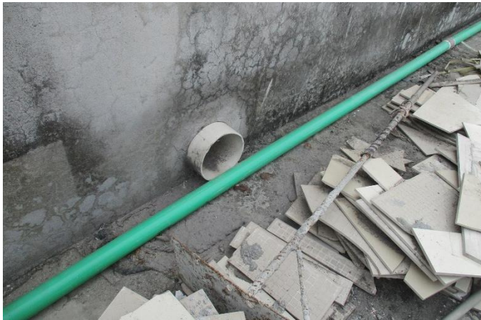
Inactive water outlet, 50 mm above roof level
