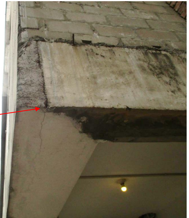
Crack in cantilever beam edge
