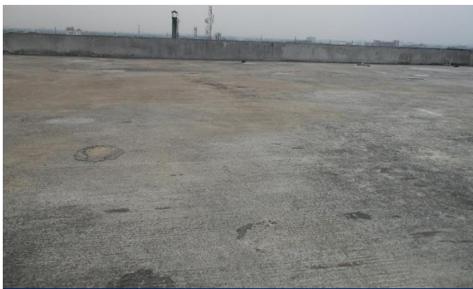
Sign of water ponding on roof slab
