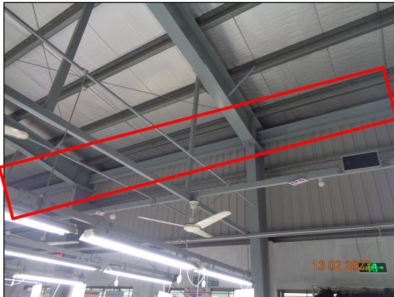
Compression Strut – Marked location
