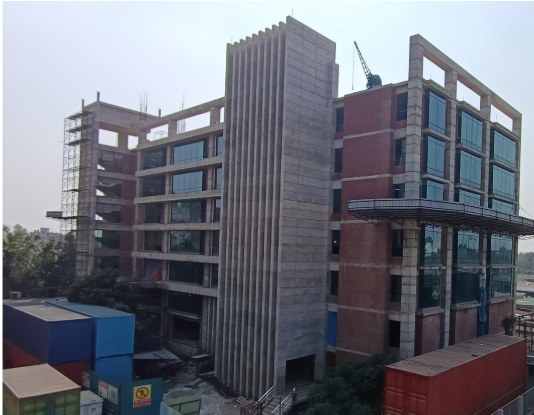
No design report was available for Production Building-2
