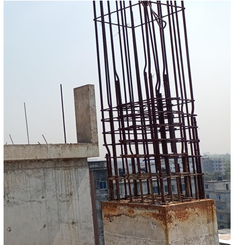
Exposed rebar at column on roof
