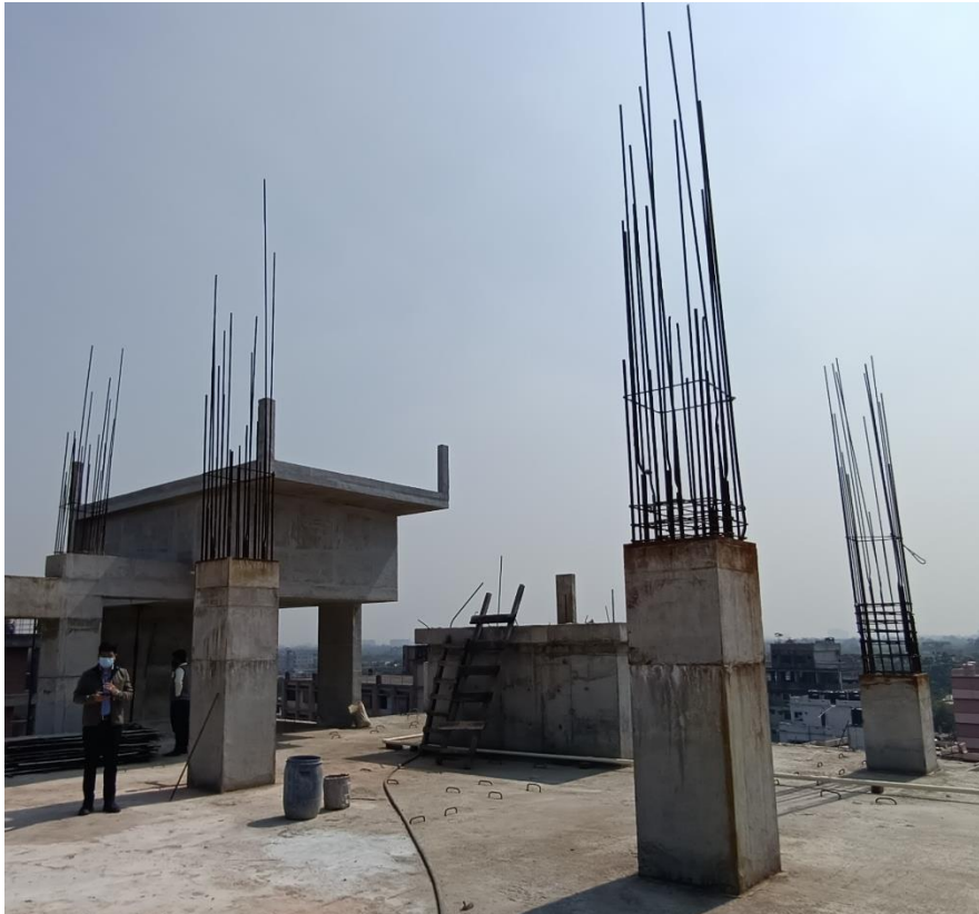
Exposed rebar at column on roof
