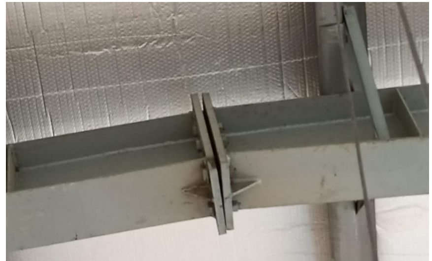
Gap observed in rafter connections
