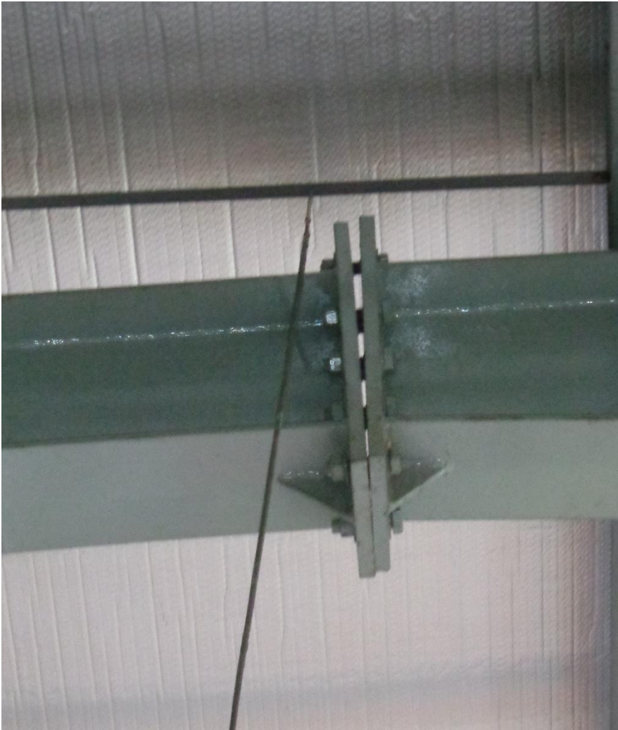
Gap observed in rafter connections
