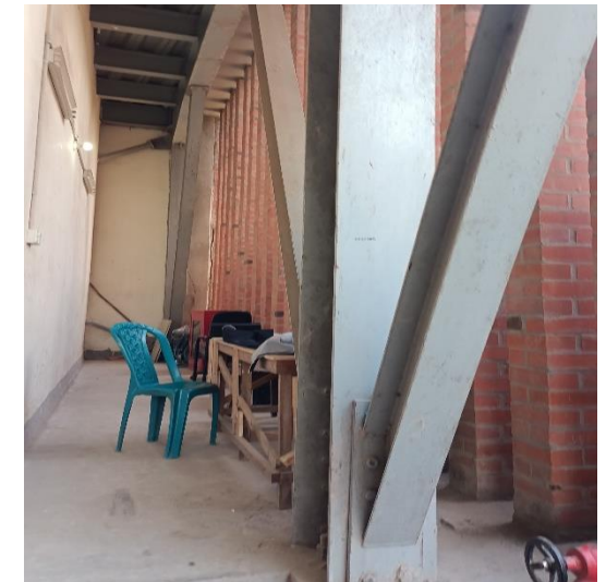
Connection of vertical bracing
