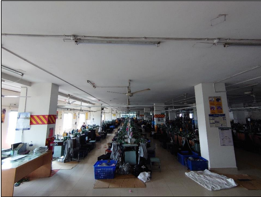
RC column and flat plate system
