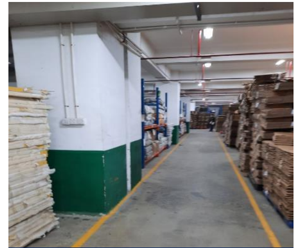
Basement column susceptible to trolley impact
