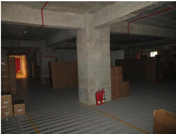
Storage on mezzanine floor
