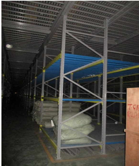
Bracing in rack frame
