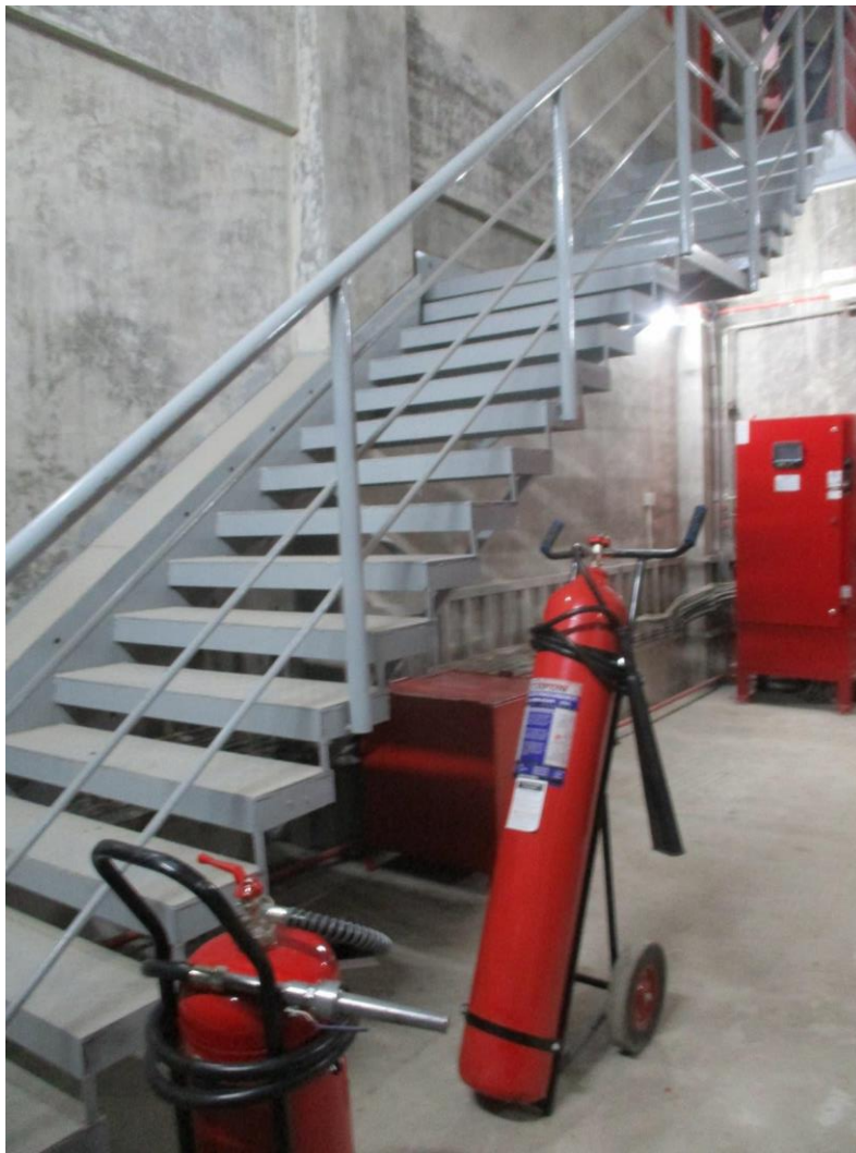
Steel stair connected with the retaining wall of basement floor
