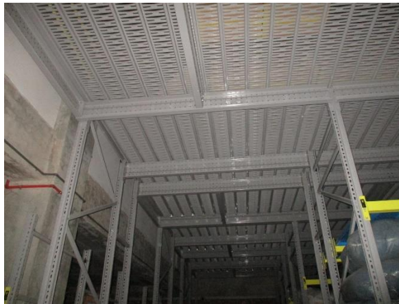
Roof system of mezzanine floor
