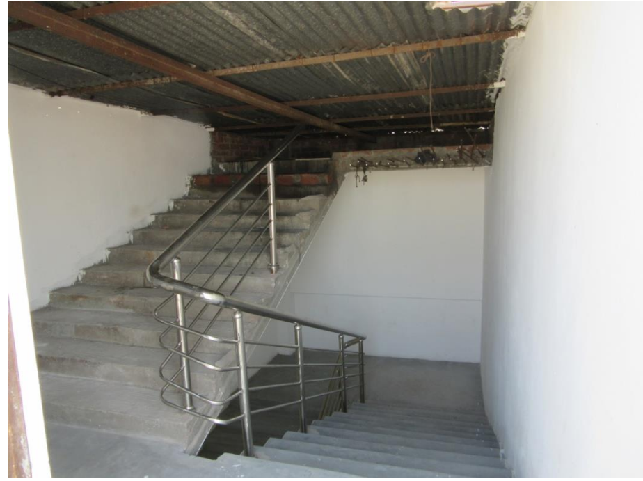
Stair at level 7
