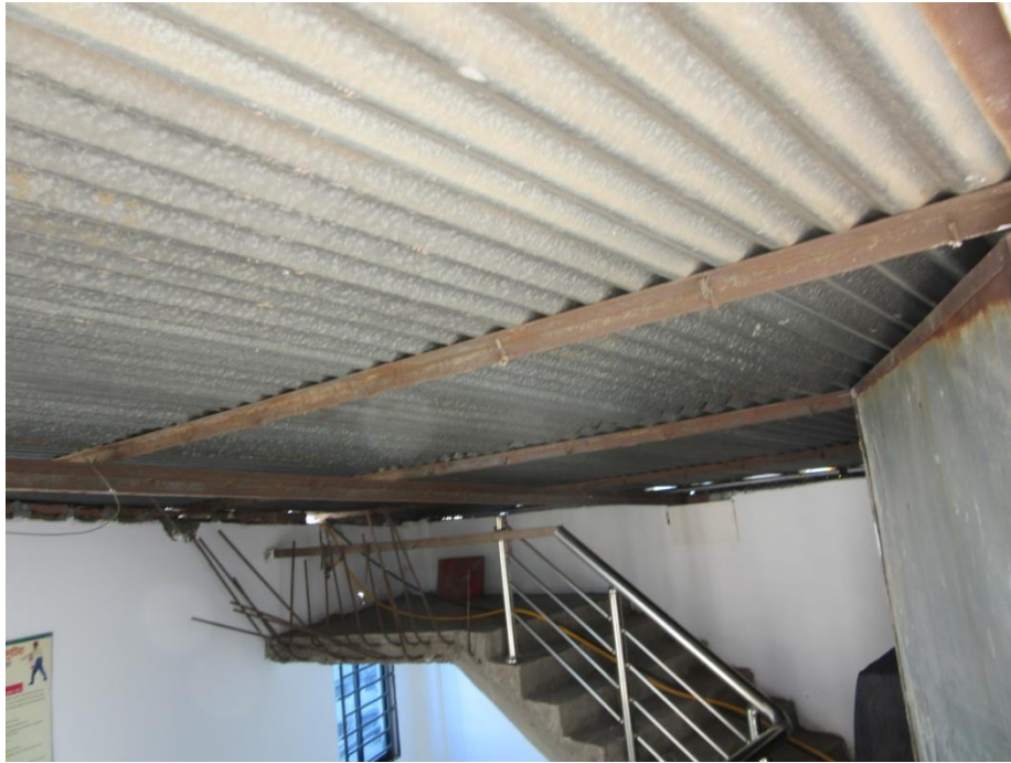
Stair near canteen at level 6
