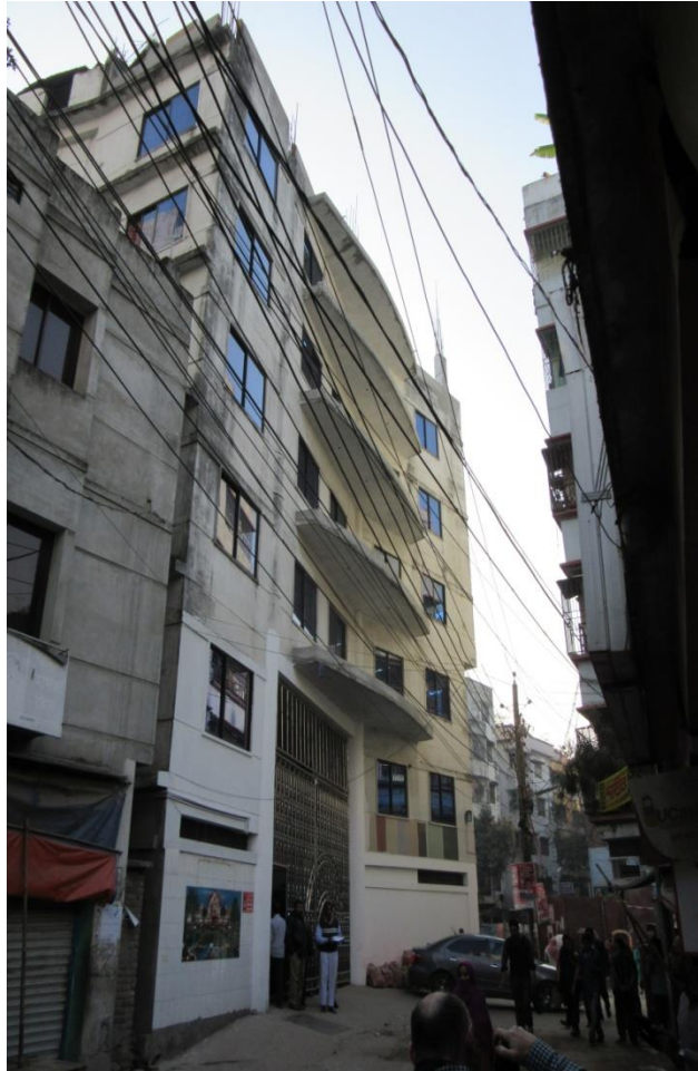
Cantilever at West side
