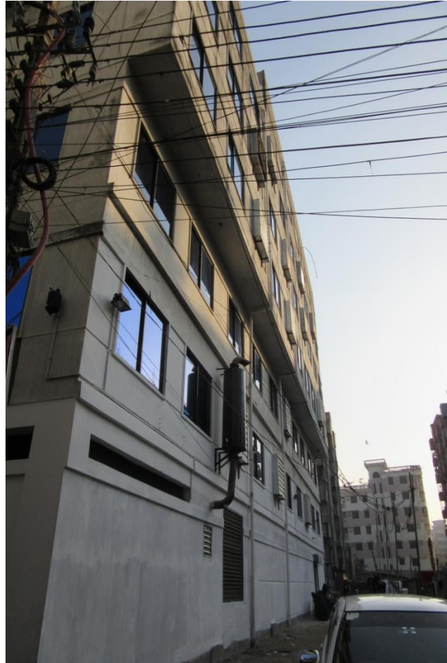
Cantilever at south side
