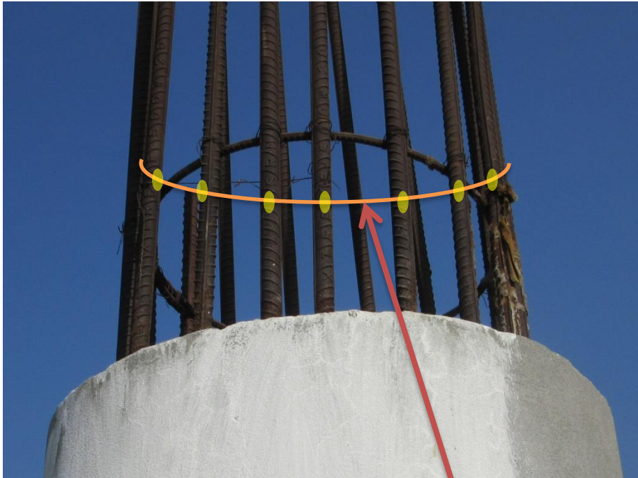
Rebar Fabrication found on site
