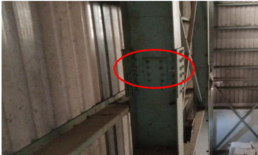
Connection gap in joints
