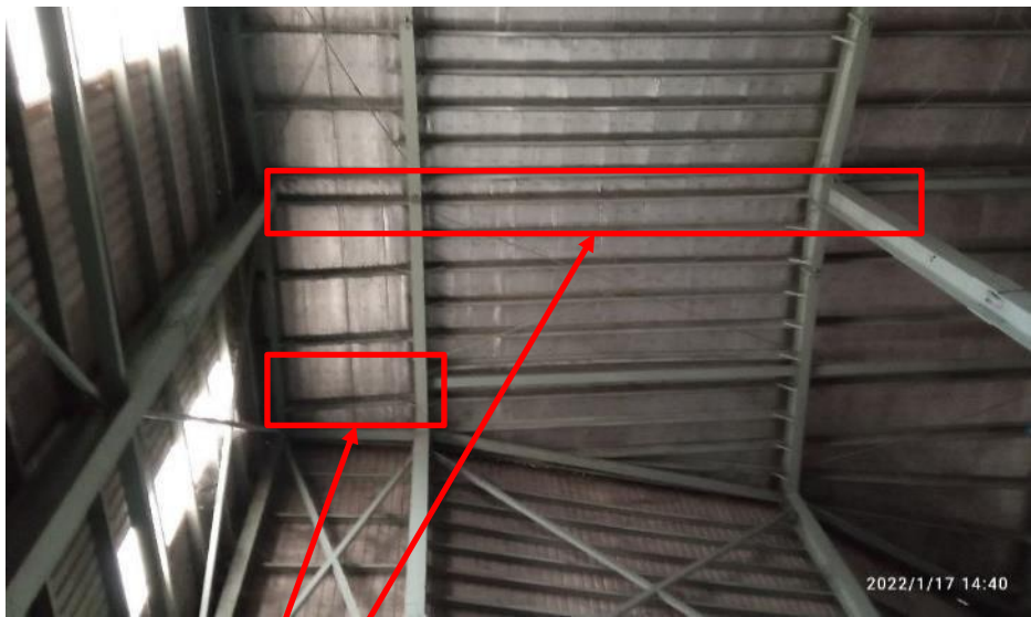
Missing compression strut on roof
