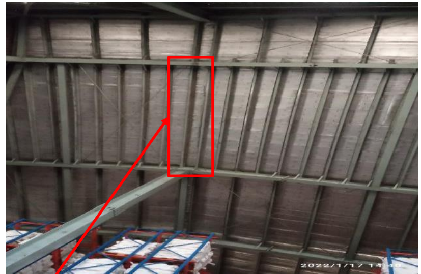
Missing compression strut on roof
