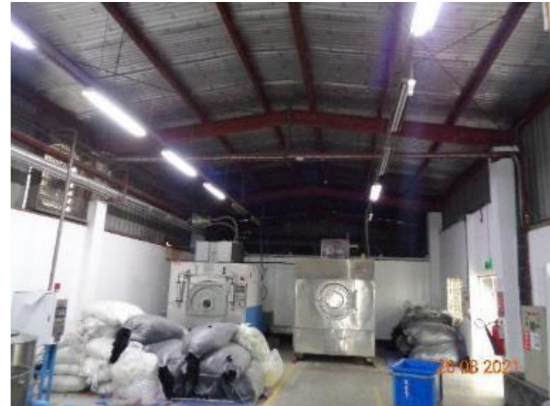
Absence of load transfer media in long direction
