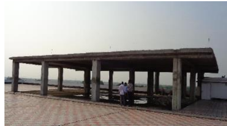
Additional roof extension
