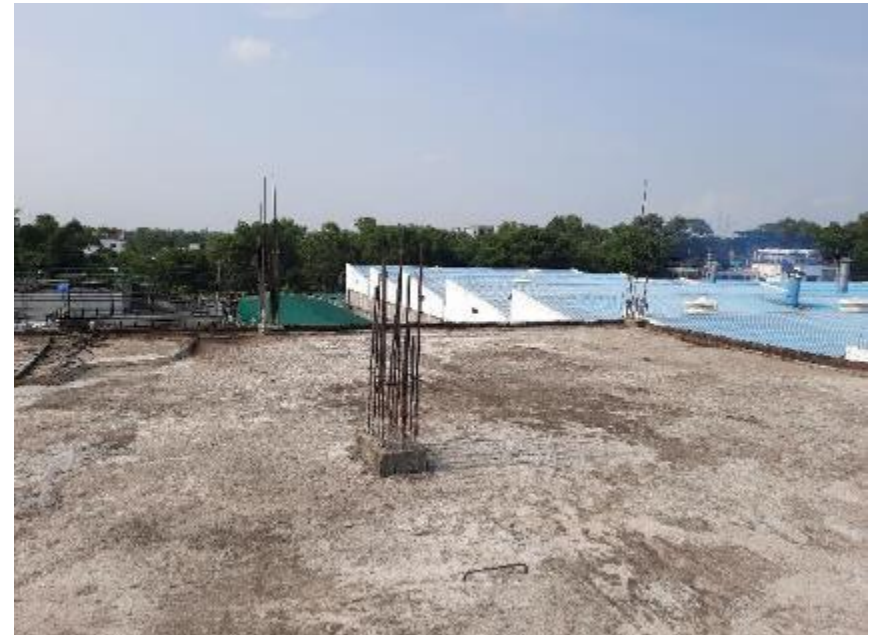
Exposed rebar indicated further construction
