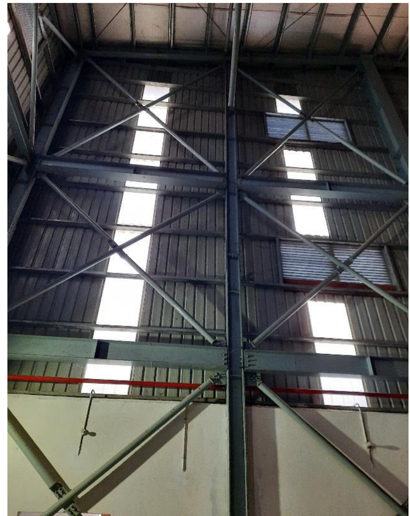
Bracing System on site
