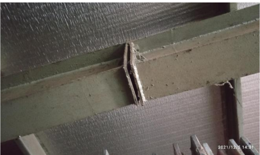
Connection gap at rafter joints
