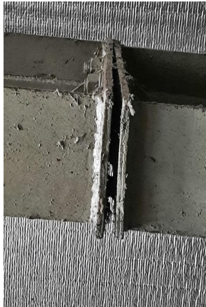
Connection gap at rafter joints
