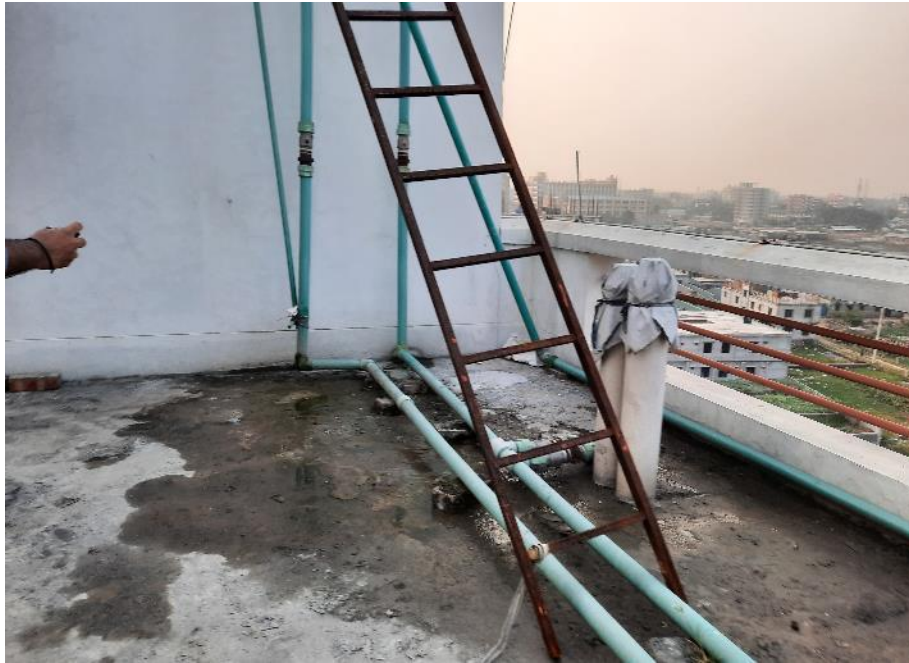
Stagnant of water observed on roof. Building engineer is required to improve the roof drainage system.
