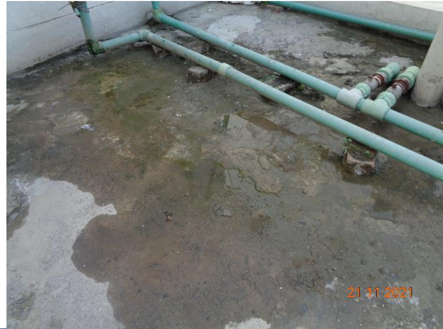
Stagnant of water observed on roof. Building engineer is required to improve the roof drainage system.
