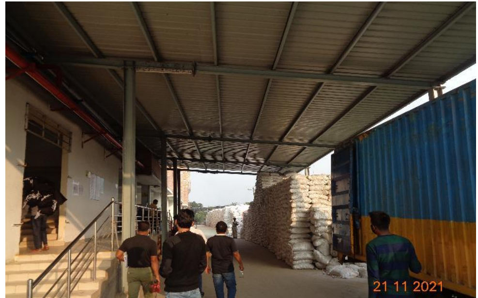
Undocumented loading unloading porch
