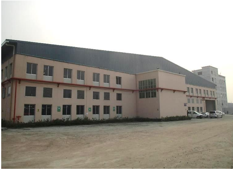
Building-1 (Steel Building)
