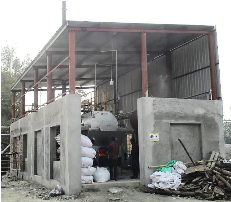
Steel framing without bracings
