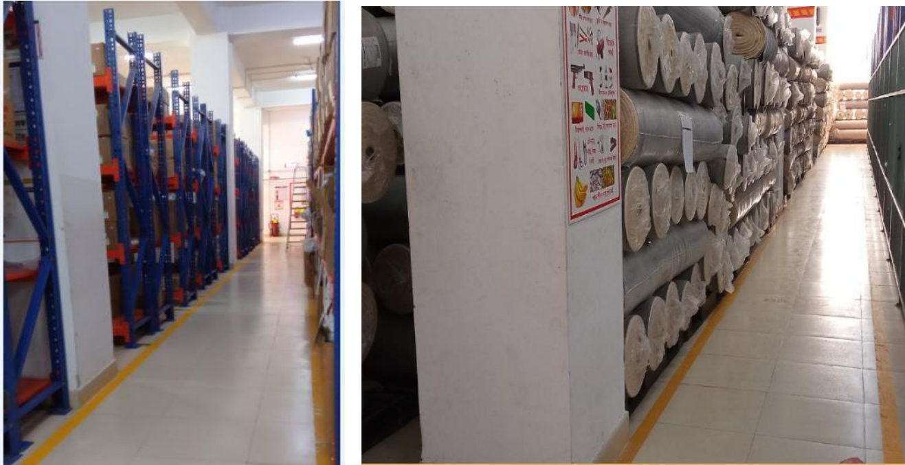
Column susceptible to trolley impact
